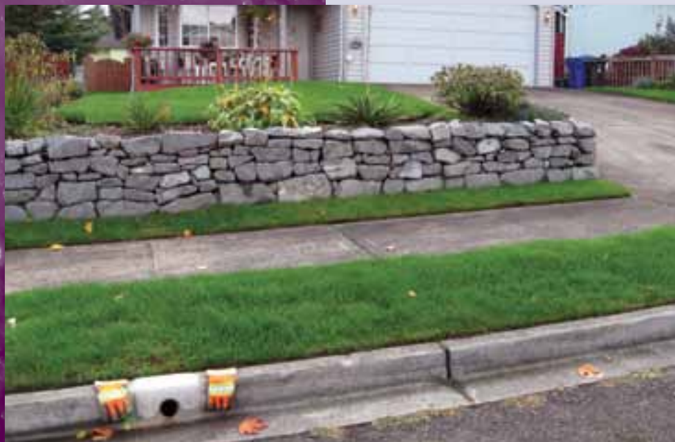
Direct downspouts to at least 10 feet away from your home or business's foundation. This can be done with "flex pipe" (shown above) or a "curb cut" (shown below).
