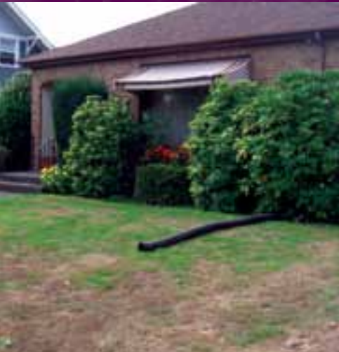
Direct downspouts to at least 10 feet away from your home or business's foundation. This can be done with "flex pipe" (shown above) or a "curb cut" (shown below).
