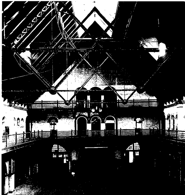
The exposed metal roof-truss system of this waiting room not only provides structural support, but is also important in defining the interior character of the train station.
