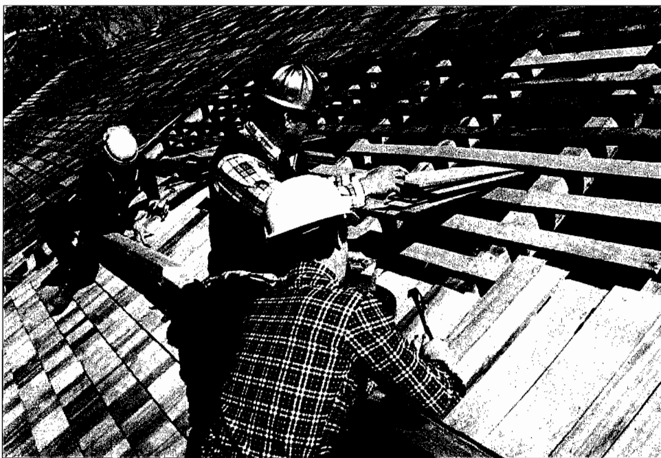
The size, shape, and detailing of the historic shingles as well as the method of fabrication and installation were carefully researched prior to selecting this new wood-shingle roofing.
