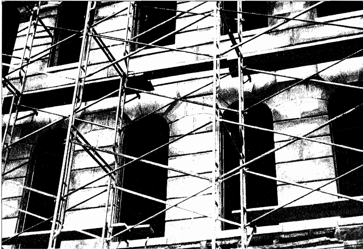
Composite patching with a cementitious mixture is being used to repair eroded areas of this sandstone facade.
