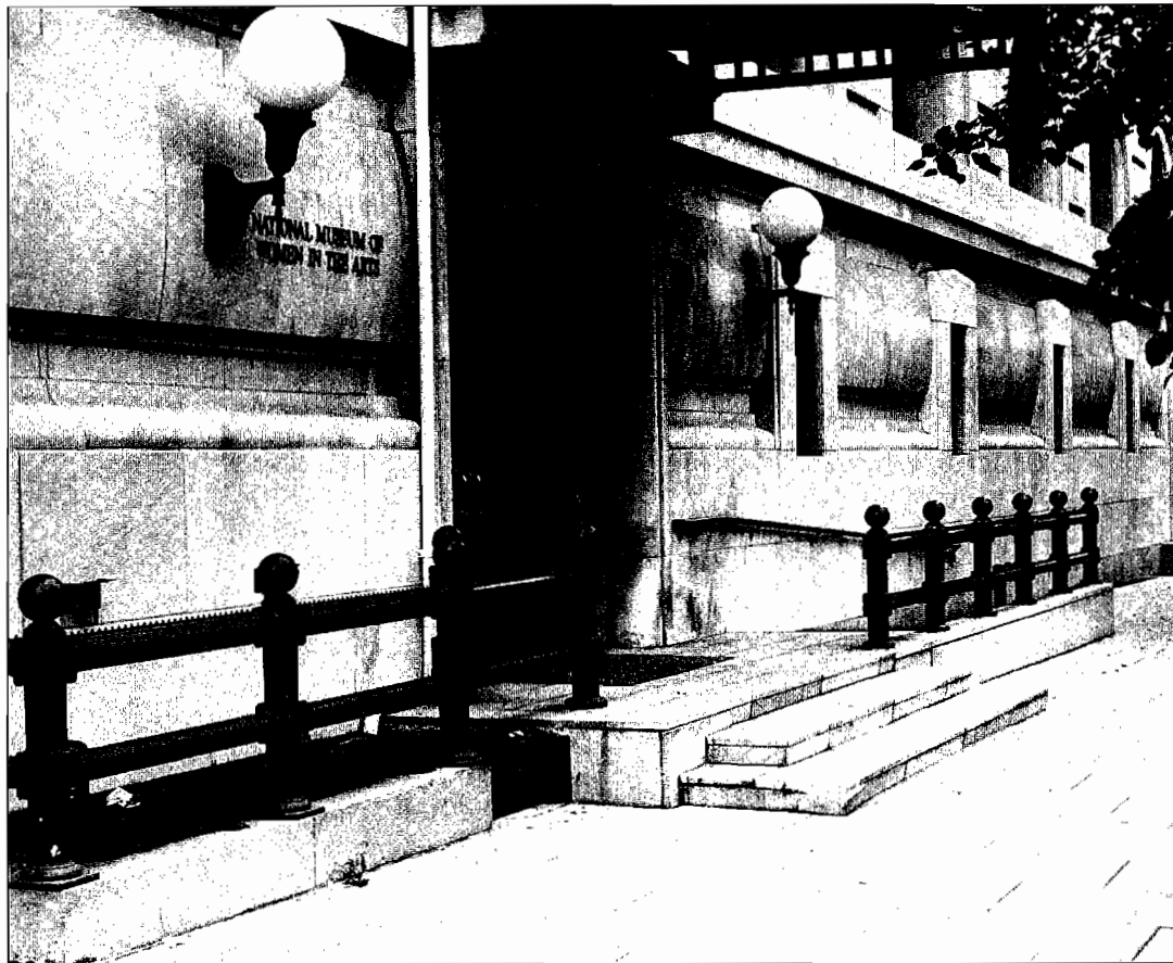
The historic cast iron railing was preserved when a permanent ramp was designed for this museum's main entrance.
