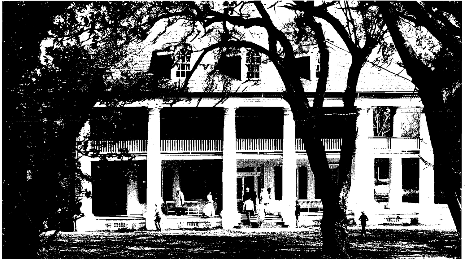
In hot climates, buildings were historically designed to minimize the heat gain from the summer sun. The wide roof overhangs, exterior porches, shutters, shade trees, and heavy masonry walls (painted white) are all energy saving characteristics.
