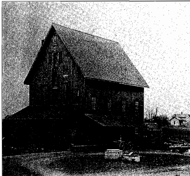
The stream and circular wagon approach are important features of this historic mill site.
