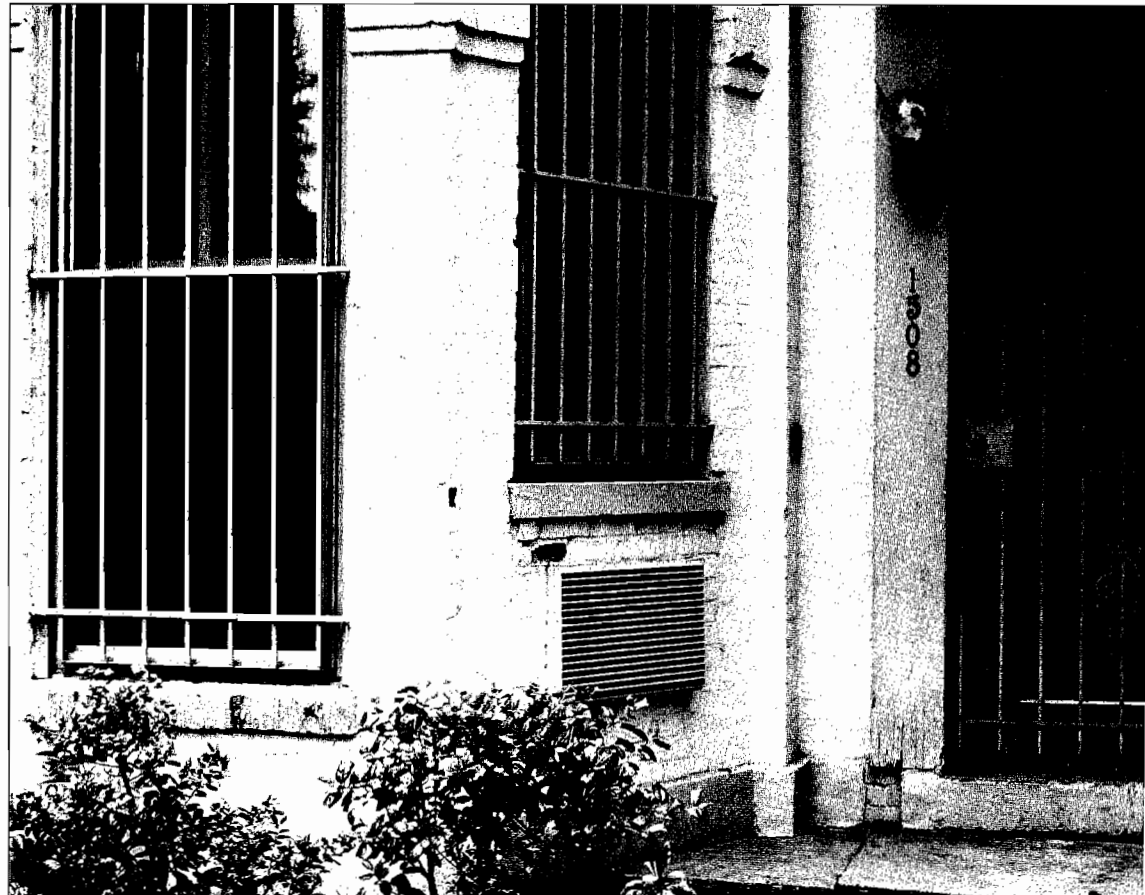
The historic window on a primary facade has been shortened and the area below it filled in with brick in order to install a through-the-wall air conditioning unit. In addition to changing the window size and destroying the sill, the unit itself is visually obtrusive.
