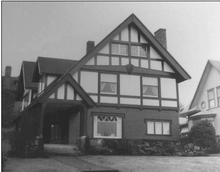
Tudor Revival house at 702 North I Street Photo courtesy of Tacoma Public Library, BU 601
