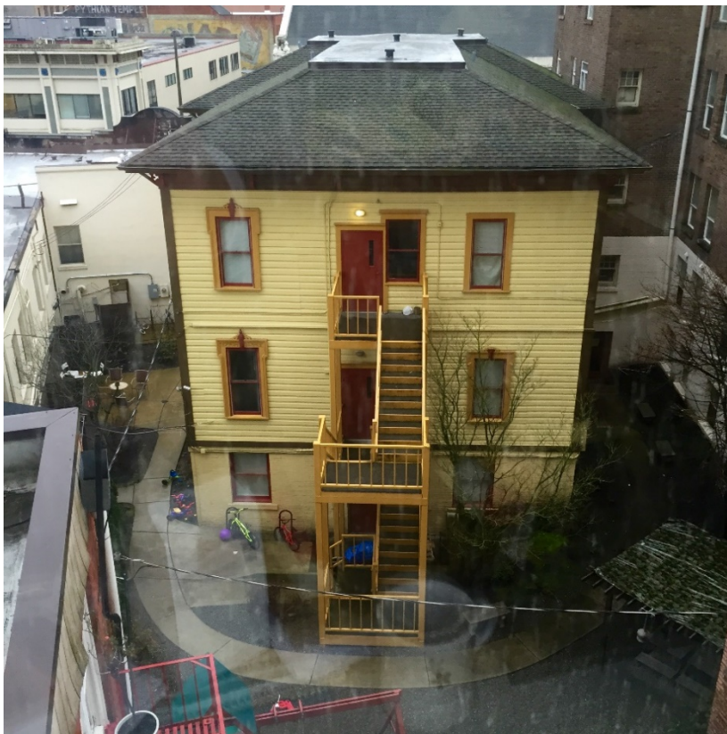
Fig. 4. North rear façade. 2015. Source: McKnight
