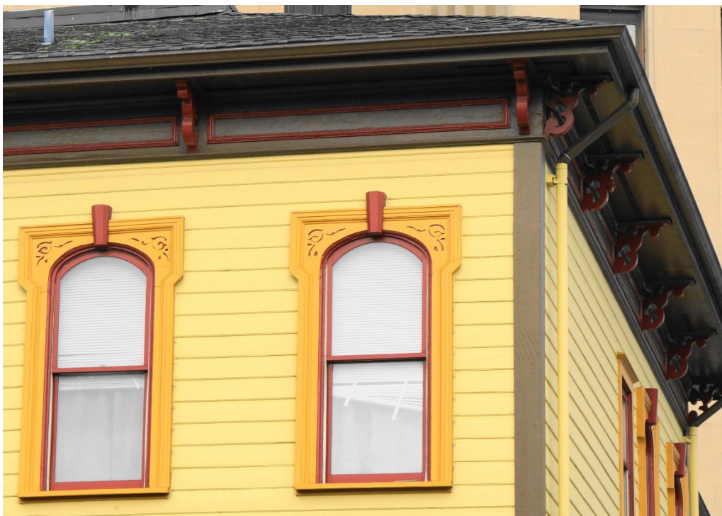
Fig. 2. Front south façade. Cornice and window detail. 2016. Source: Erikson
