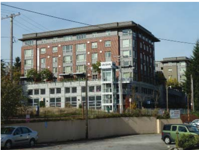
FIG. 9-13 The Court 17 apartments are built above three levels of parking managed by the UWT .
