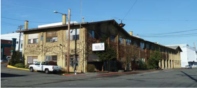
FIG. 11-16 The City Streets and Grounds Building, view from South C Street.
