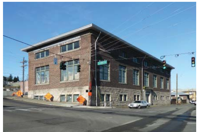
FIG. 6-8 The 1911 Nisqually Power Plant substation at 2416 South C Street.
