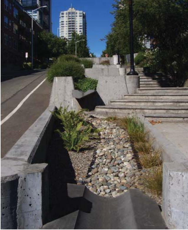
FIG. 8-13 This artful stormwater conveyance system is part of a community garden in Seattle’s Belltown neighborhood.
