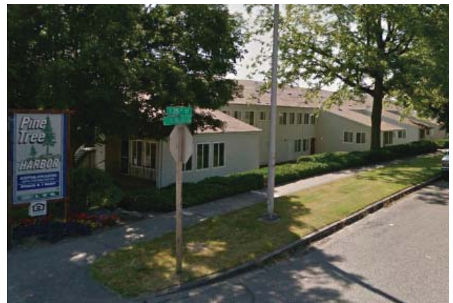
FIG. 5-10 Pine Tree Harbor Apartments at 2501 South G Street (Trieste Holdings)
