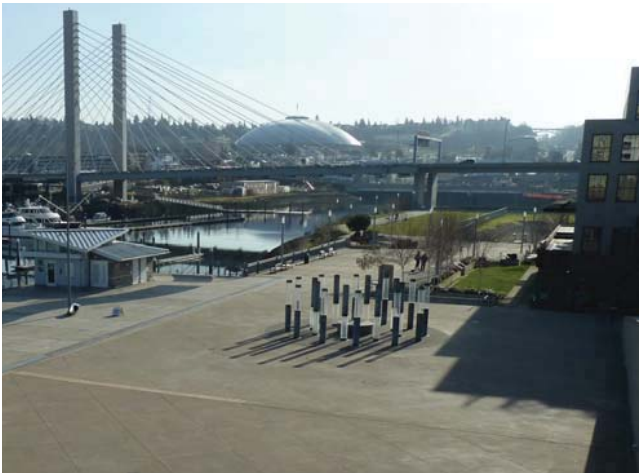
FIG. 8-6 The Foss Waterway Esplanade provides a continuous public walkway along South Downtown’s waterfront. When complete, it will stretch 1.5 miles from the head of the Thea Foss Waterway to its end.
