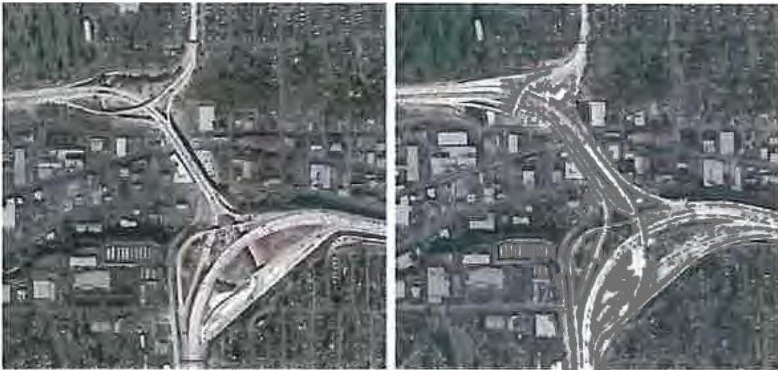
WASHINGTON STATE DEPARTMENT OF TRANSPORTATION - An aerial view of the westbound Interstate 5/state Route 16 interchange construction in Tacoma taken in December 2010, right, shows the dramatic changes that have taken place since the project began in the Nalley Valley 2009. The photo at left was taken in October of 2005. The first phase of the project is scheduled to be completed next summer. Order News Tribune reprints Order Associated Press reprints
