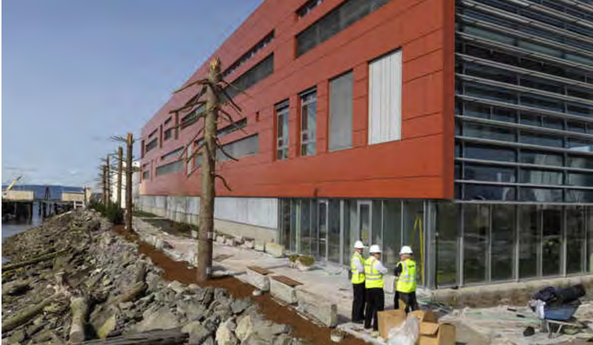
Staff photographer - The Center for Urban Waters on Tacoma's Thea Foss Waterway is a model of green design and construction. Features shown here include fixed sun shades on the south side, right, and exterior venetian blinds on the west side.
