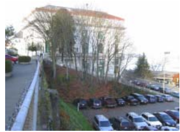
CP. 5.2.19 View looking north at the south slope.
