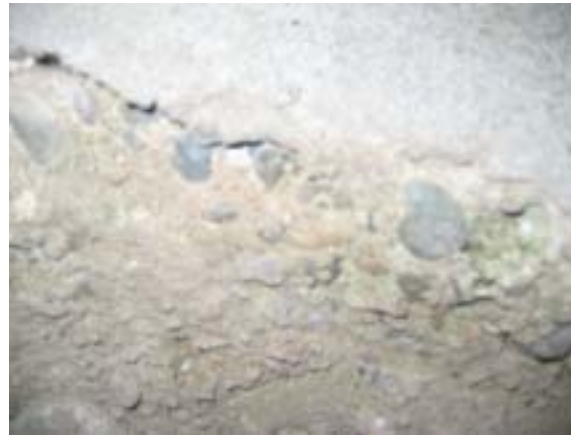
CP. 5.2.21 Detail view of underside of retaining wall.
