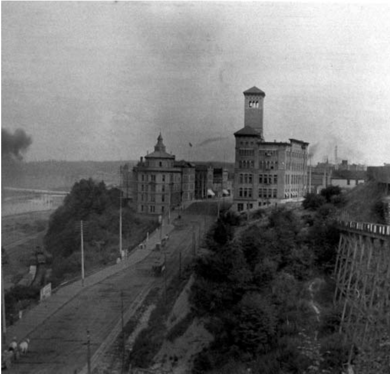
ca 1895 photograph of Pacific Avenue looking south. Source: Washington State Historical Society.
