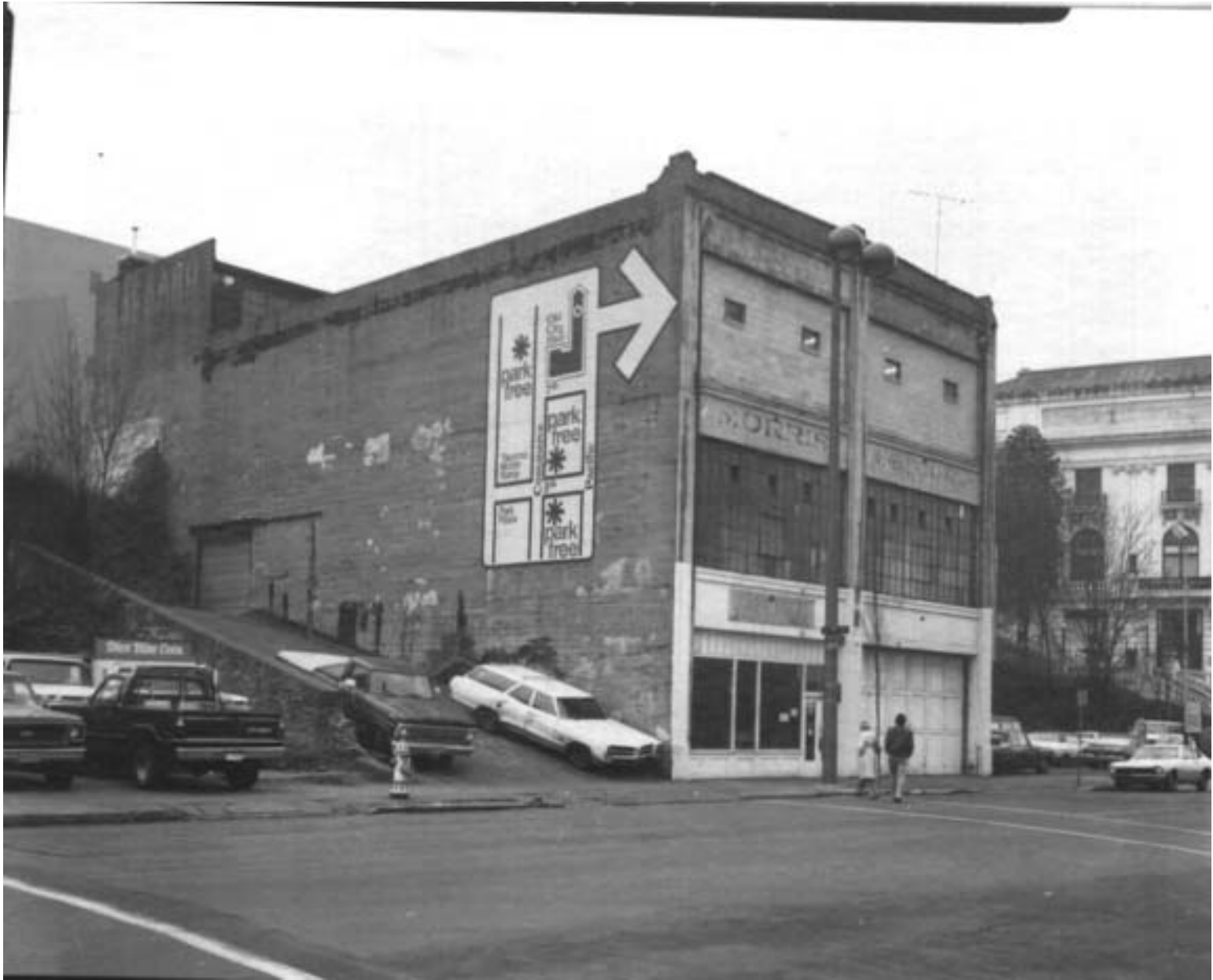
1977 photograph of the former building in the adjacent south lot. Source: Old City Hall National Register Historic District Nomination (1977).
