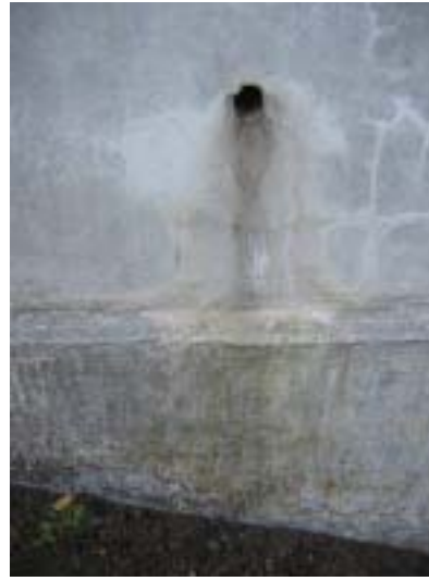
CP. 5.2.12 Weep hole in a typical newel.
