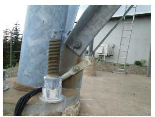
037 Capitol Peak Corrosion, Spalling Grout
