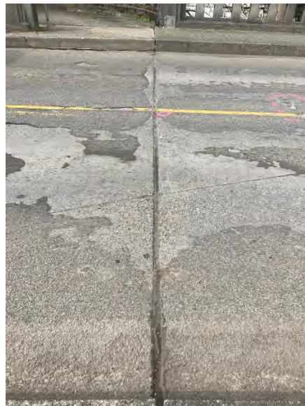
Failed construction joint with associated delaminations
