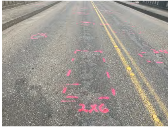
Typical delamination in wheel line
