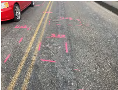
Delamination inside wheel lines
