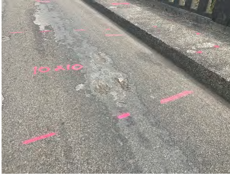
Delamination, spalls, and exposed reinforcing steel.
