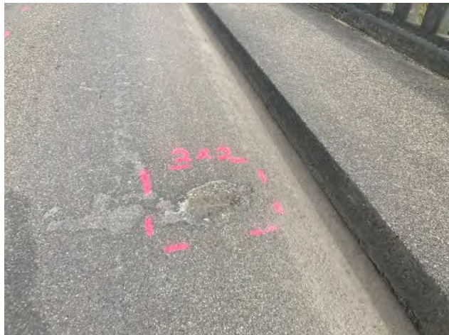
Deck delamination with exposed reinforcing steel
