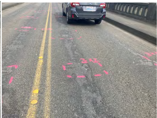
Deck delamination with exposed reinforcing steel
