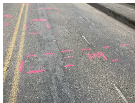
deck cracking with delamination
