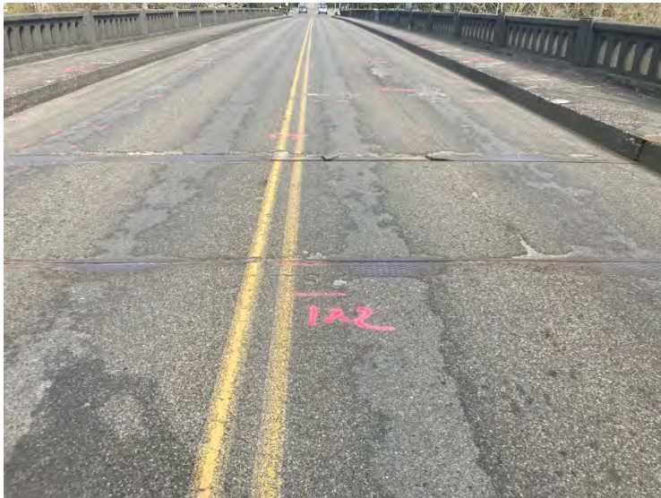
Failed expansion joints with delaminations
