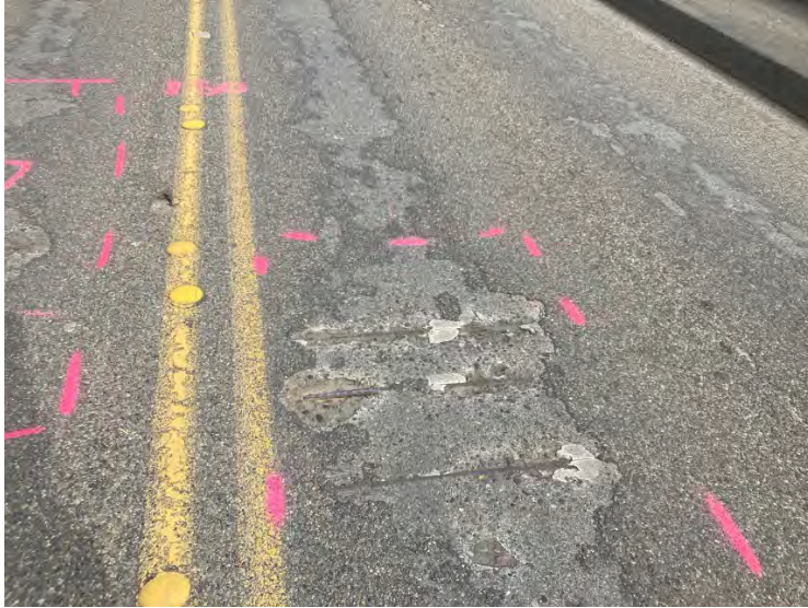
Delamination with exposed reinforcing steel
