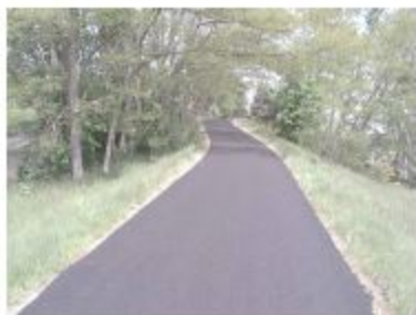
TRAIL - BUILT TO STANDARD (PHASE I CONSTRUCTION)
