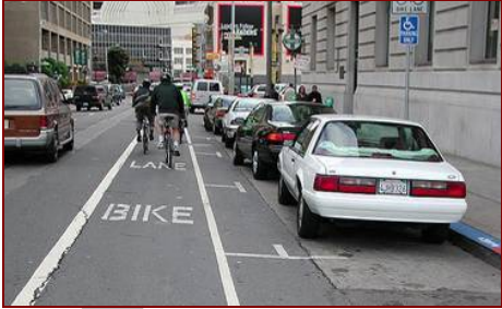
This bike lane provides parking "T"s to minimize the danger of 'dooring'
