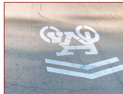
Shared lane marking
