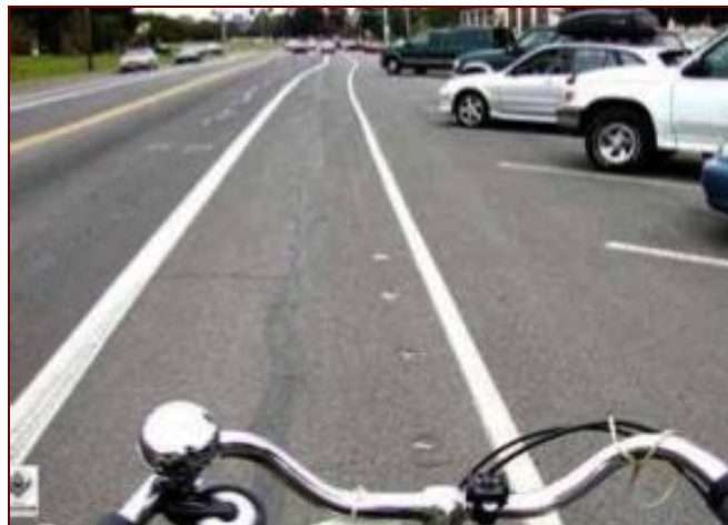
'Back-in' diagonal parking is safer for cyclists than 'head-in' diagonal parking due to visibility
