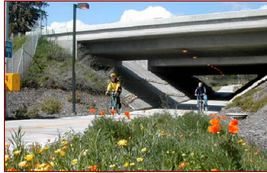
Type 4 Grade-Separated Undercrossing
