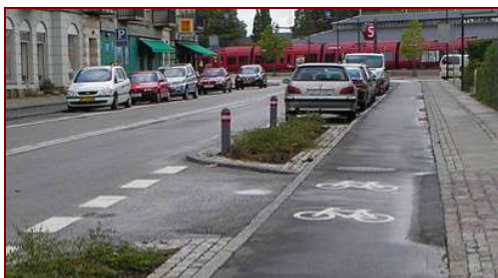
Medians, driveway consolidation, or restricted movements reduce the potential for conflict.
