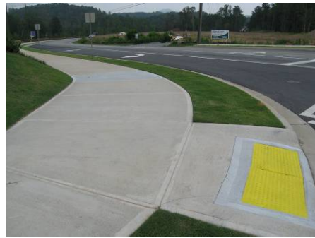
A diagonal ADA-compliant curb ramp
