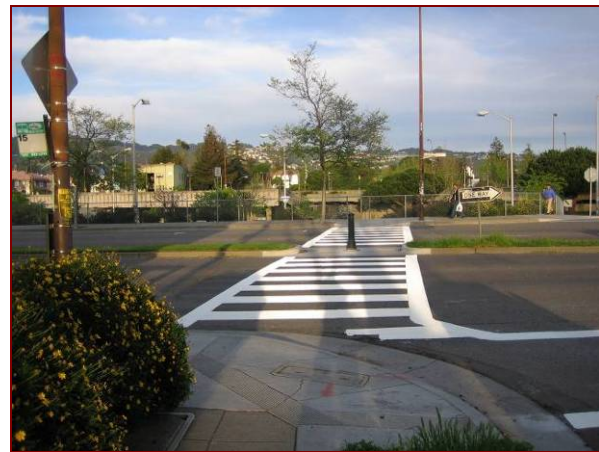
Ladder pavement markings (shown), and European type crossings are the preferred crosswalk design for Tacoma
