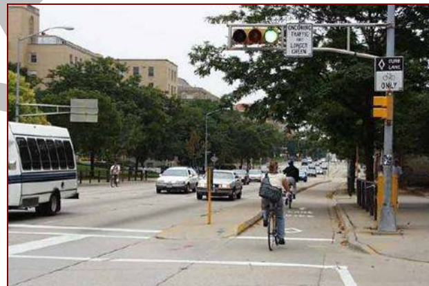
This contraflow bike lane in Madison, WI uses a physical barrier from traffic at the intersection
