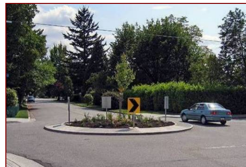
Mini traffic circles require that both bicyclists and motorists slow down and watch for conflicts
