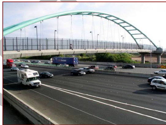
Type 4 Grade-Separated Overcrossing
