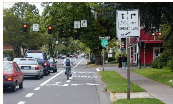
Shared bike-right turn lanes require warning signage as well as pavement markings
