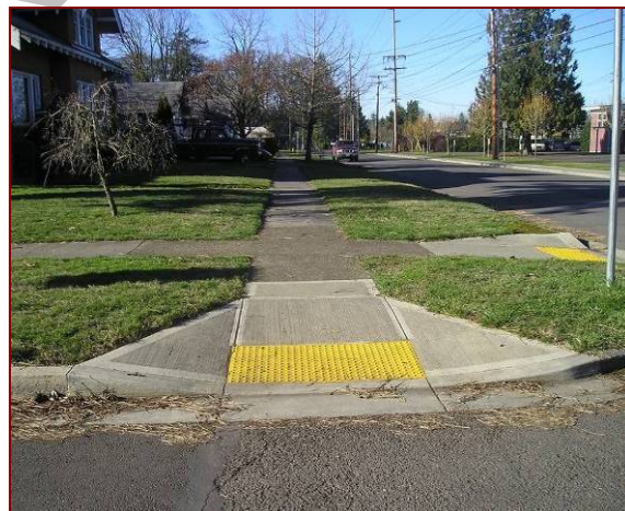
Example of an ADA-compliant perpendicular curb ramp
