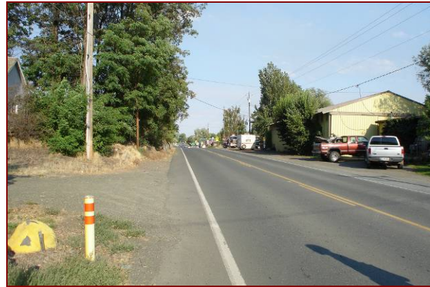
Shoulder bikeways are appropriate along wide roads where vehicles can avoid passing close to bicyclists
