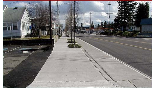
Concrete is often used as a shared-use path material, and also can be used for sidewalks
