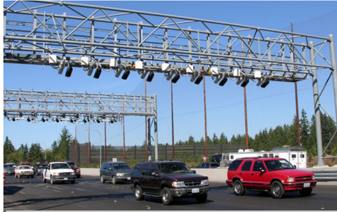
Electronic Toll lanes at the Tacoma Narrows Bridge
