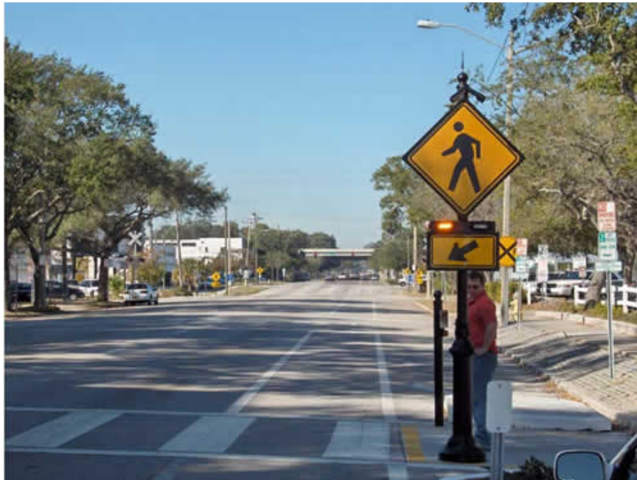
Exhibit 5. Rectangular Rapid Flashing Beacon System
