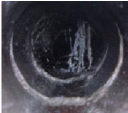
**Clean groundwater pouring in through a defective joint.**
