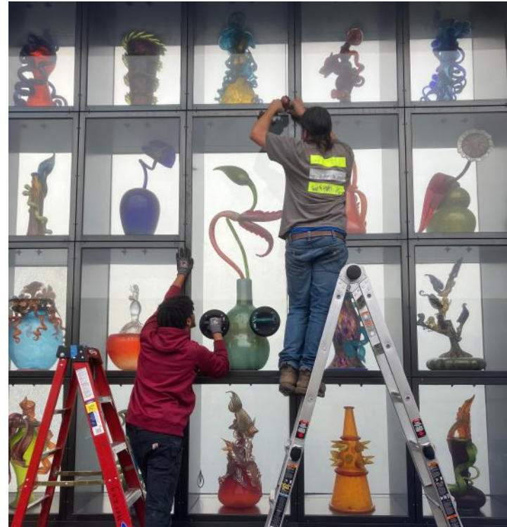
Venetian Wall panel replacement on the Bridge of Glass.
