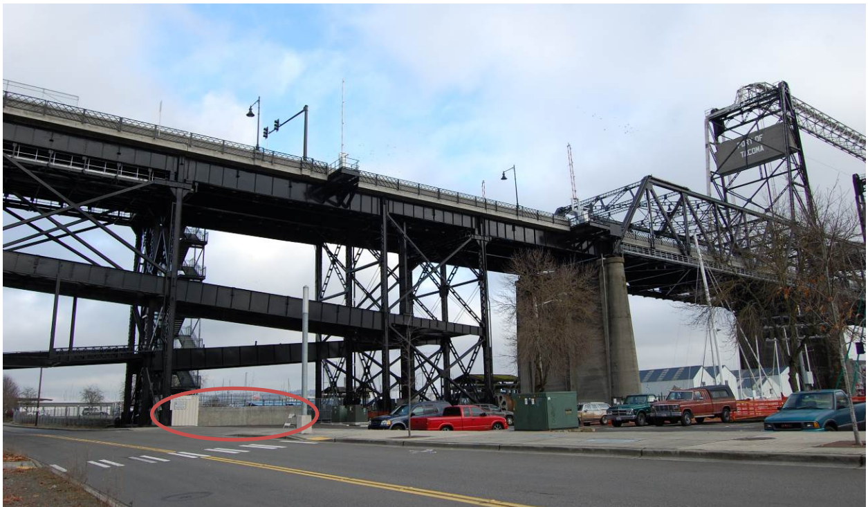
The red oval indicates the location of the stormwater collection system, located under the west side of the Murray Morgan Bridge at Dock Street and S. 11 th Street.
