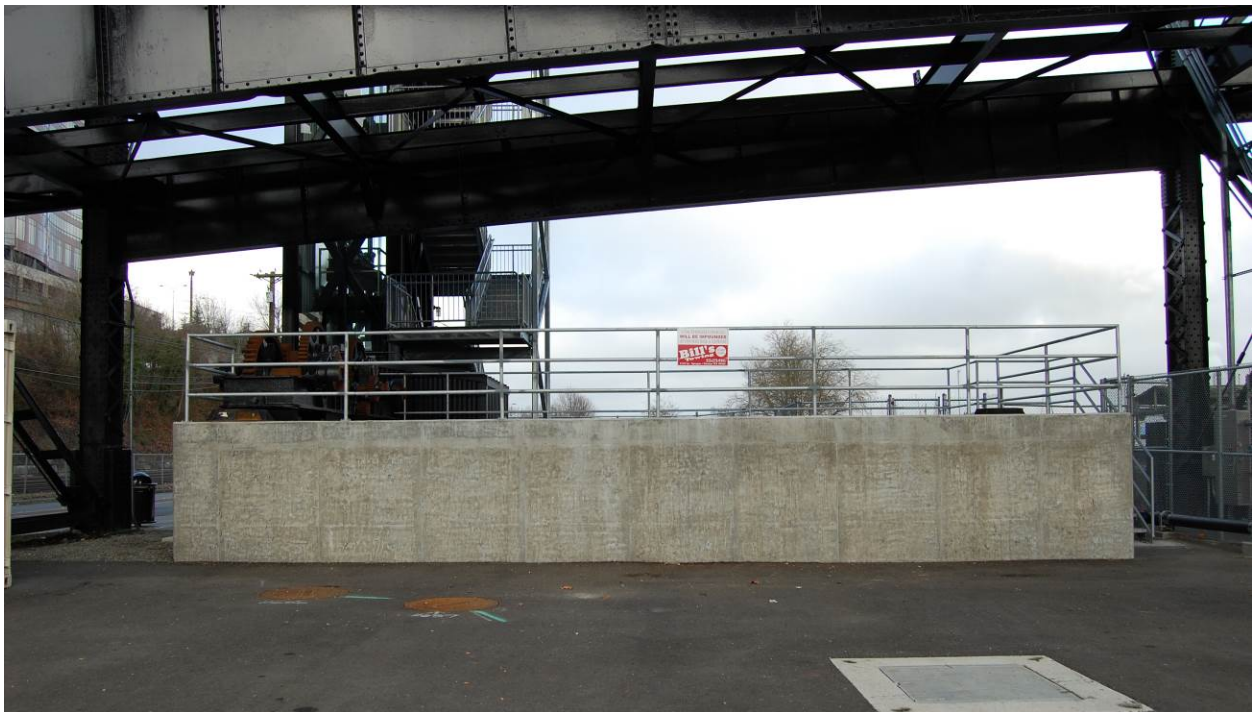
The south wall of the stormwater collection system.
