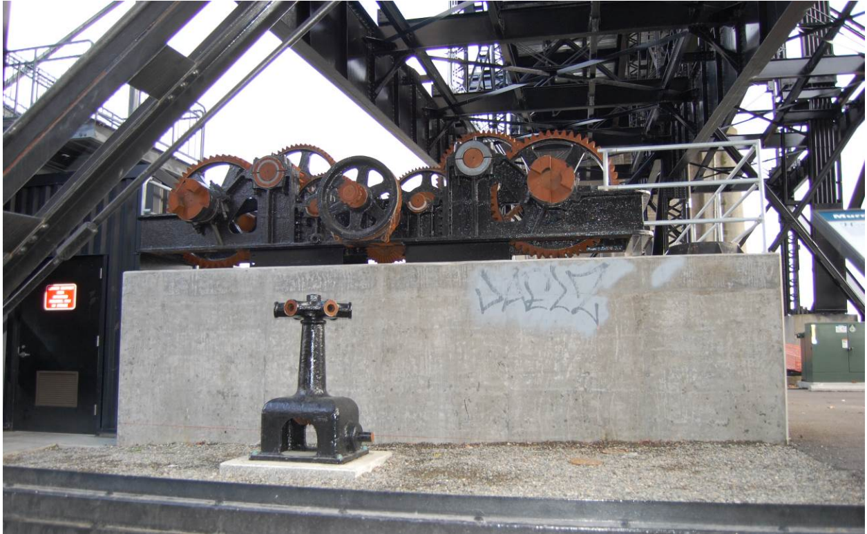
The west wall of the stormwater collection system (facing Dock Street). Mounted on top of the wall are the original gears that were used to raise and lower the bridge. The original capstan, which was used to manually raise and lower the lift span during power outages, is mounted in front of the wall.
