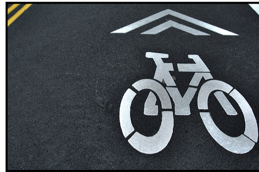
Shared Lane Marking
