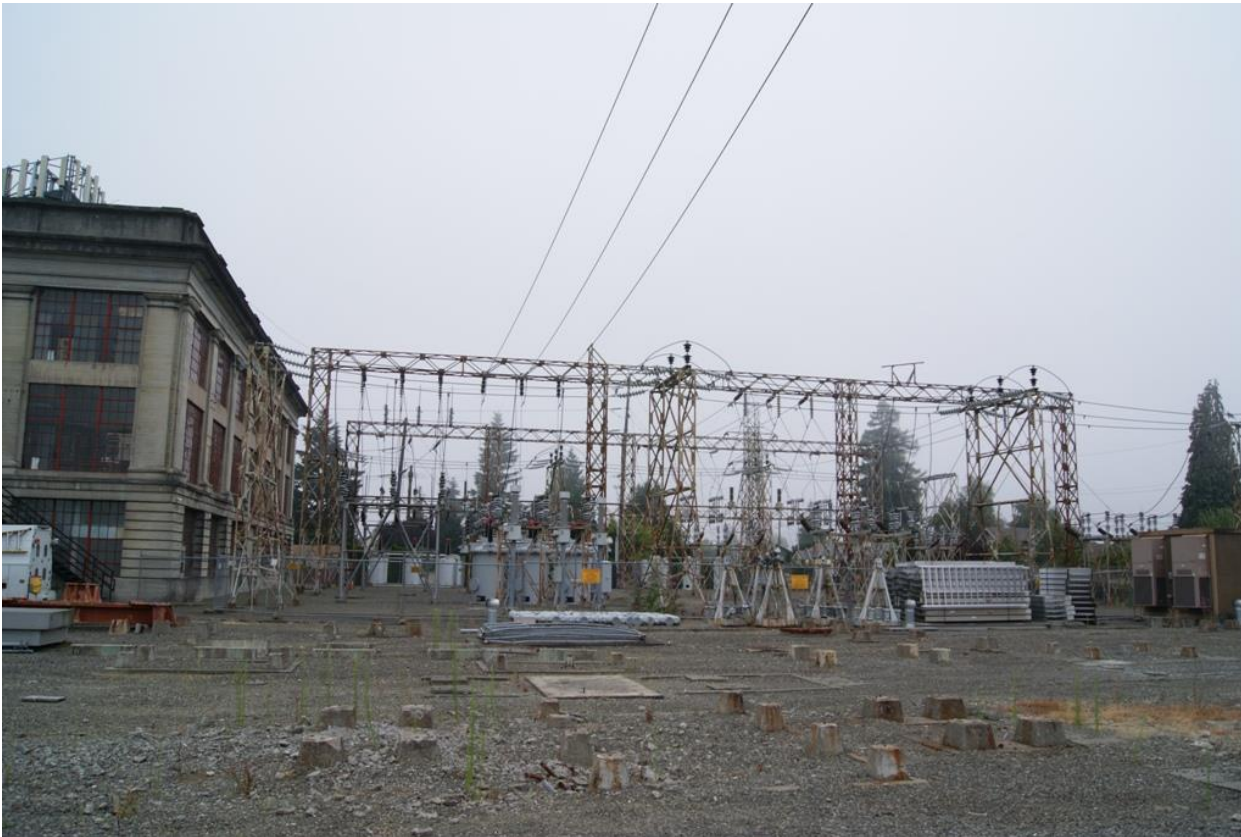
Photo 6 of 15. WA_PierceCounty_CushmanSubstation_0006. Viewing west to the exterior, modern switchyard (noncontributing) at Cushman Substation.
