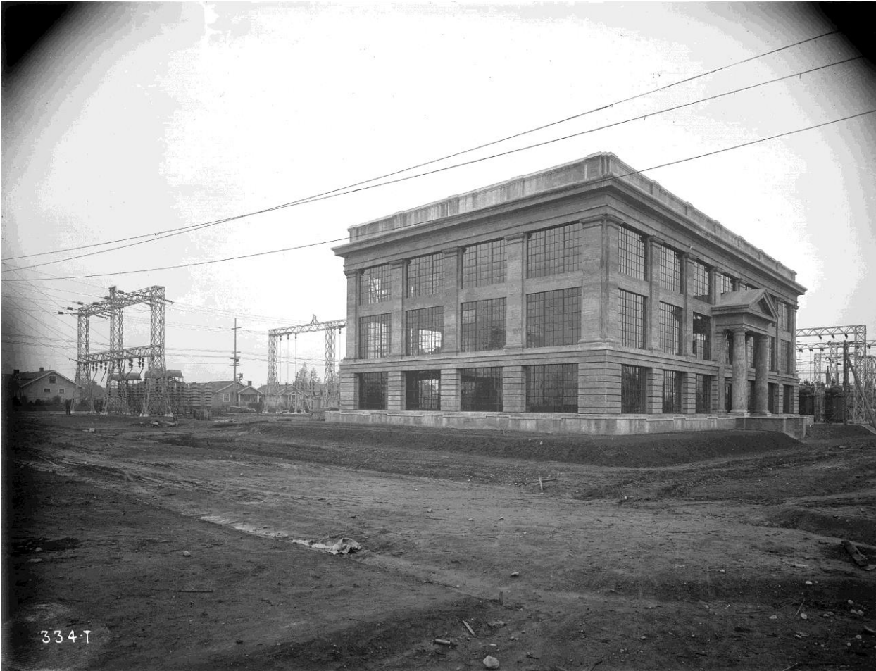
Figure 2. Cushman Substation, 1925, southwest oblique (viewing northeast) with view to switchyard. Image courtesy of Tacoma Power.
