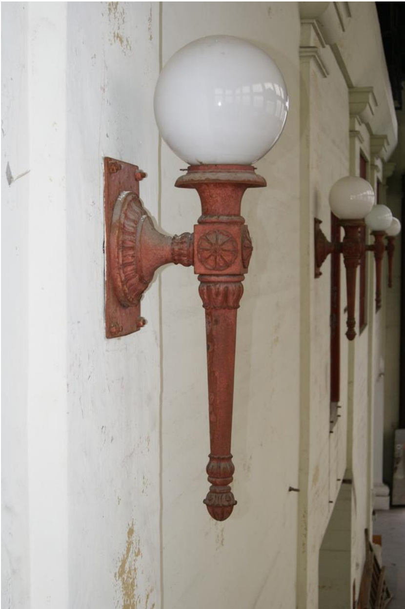
Photo 10 of 15. WA_PierceCounty_CushmanSubstation_0010. Detail of decorative light fixture at Cushman Substation.
