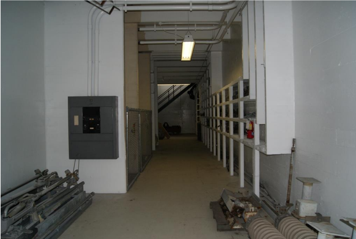
Photo 15 of 15. WA_PierceCounty_CushmanSubstation_0015. Basement level of Cushman Substation.
