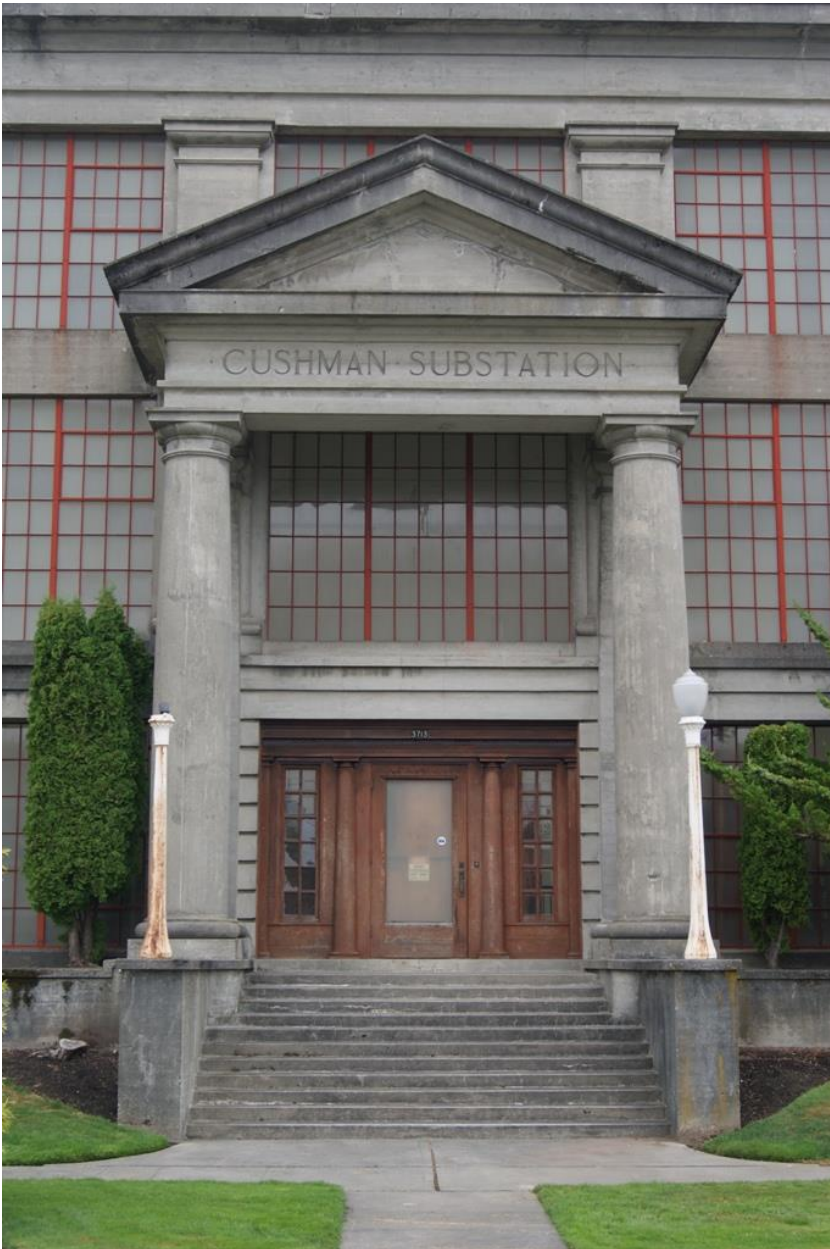
Photo 2 of 15. WA_PierceCounty_CushmanSubstation_0002. View of the temple front entrance on the façade (south face) of Cushman Substation.
