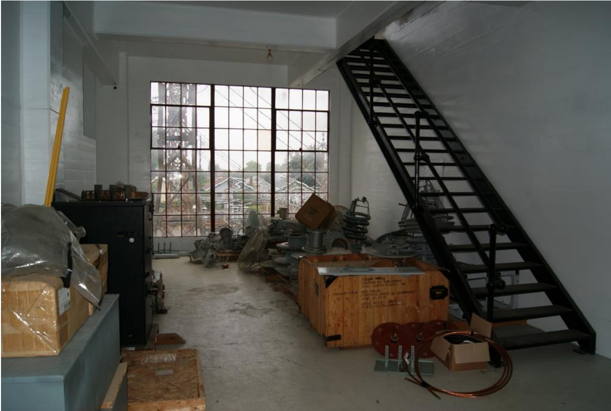
Photo 14 of 15. WA_PierceCounty_CushmanSubstation_0014. Stair from second to third level at Cushman Substation.
