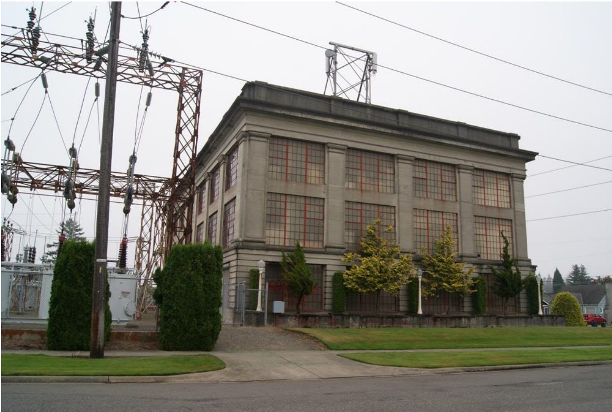
Photo 4 of 15. WA_PierceCounty_CushmanSubstation_0004. Northwest oblique of Cushman Substation, viewing southeast.
