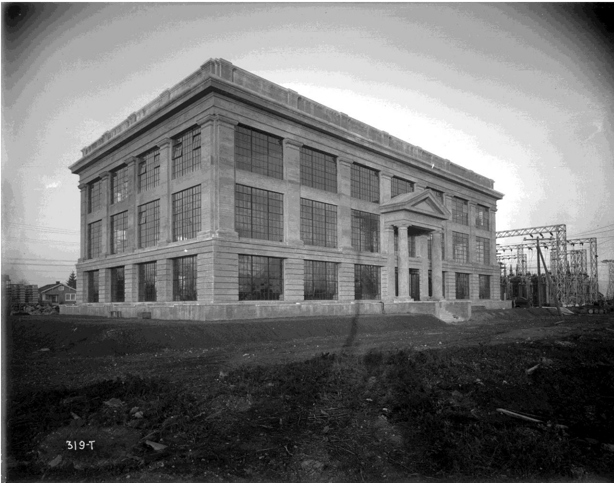
Figure 1. Cushman Substation, 1925, southwest oblique viewing northeast. Image courtesy of Tacoma Power.
