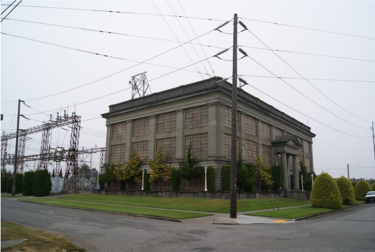
Photo 3 of 15. WA_PierceCounty_CushmanSubstation_0003. Southwest oblique of Cushman Substation, viewing northeast.
