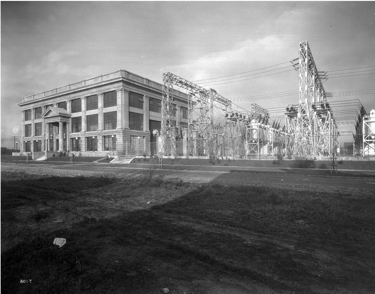
Figure 3. Cushman Substation, 1925, southeast oblique (viewing northwest) with view of switchyard (no longer extant). Image courtesy of Tacoma Power.
