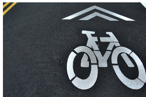
Shared Lane Marking
