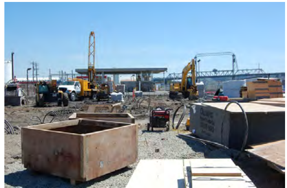
Installation of the geo-thermal wells
