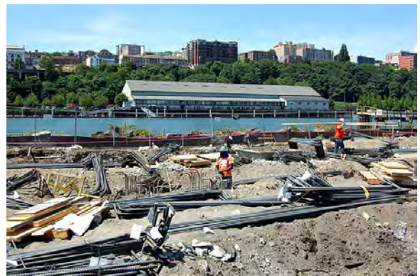
Laborers work on installing grade beam rebar
