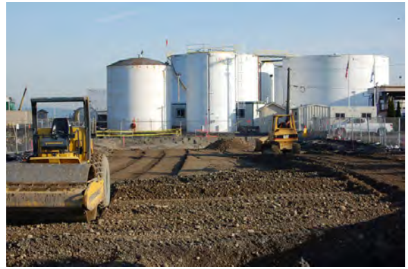
Mass excavation nearing completion
