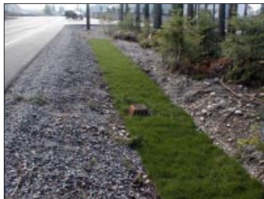
Grass lined channel: providing a filter
