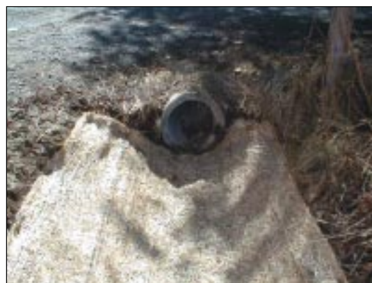
Lining a ditch with soil stabilization matting to reduce erosion
