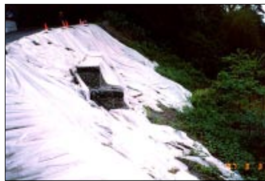
Plastic covering used to protect exposed surface from erosion during construction/repair activities
