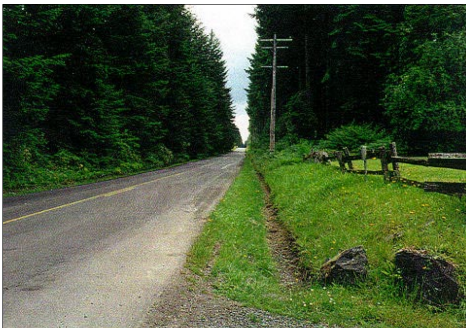
Roadside ditch with a vegetative buffer
