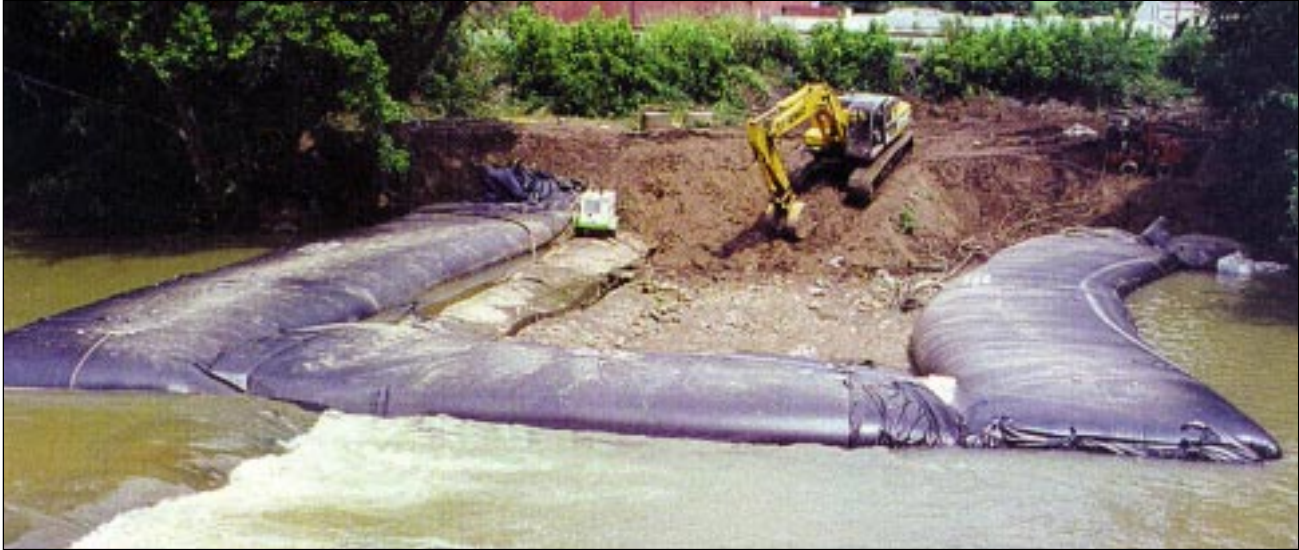
Aqua barrier used as coffer dam
