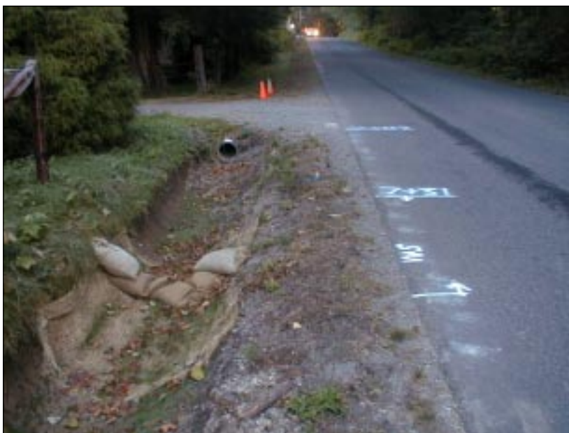
A sandbag barrier used to decrease water velocity. Note use of silt mat and hydroseeding to decrease erosion and to increase vegetation in channel
