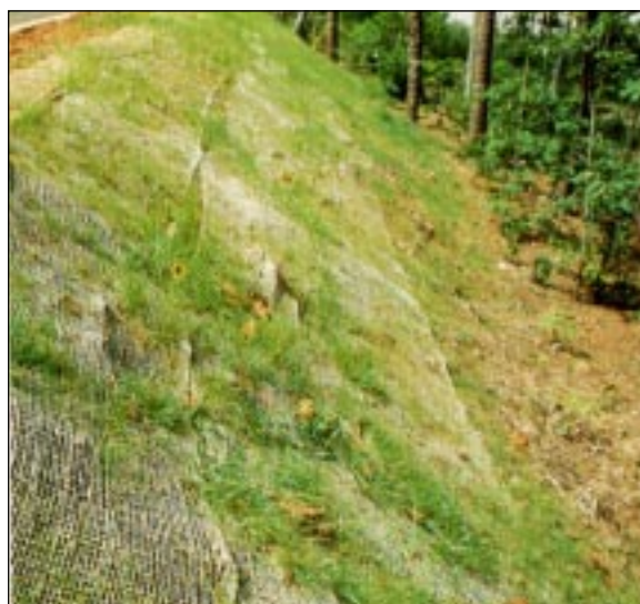
Stabilizing the soil using matting and hydroseeding
