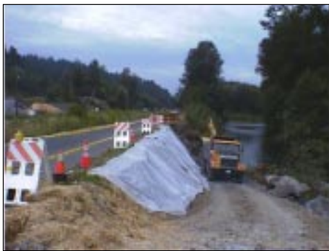
Plastic covering used as erosion protection on a slope at construction/repair area. Note additional use of mulch in area
