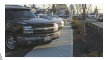
Provide wheel stops or a wider sidewalk to remedy the encroachment into the PAR.
