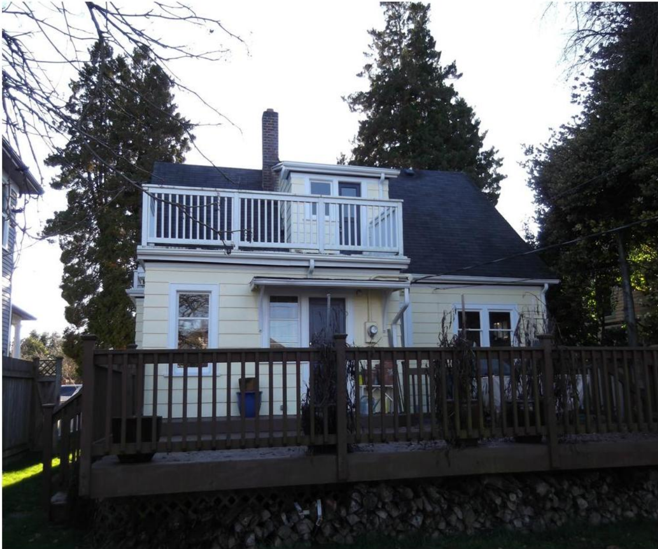
View of East area. Clarifies the replacing of the lower East door to a half lite door matching look and flow of second story door.
