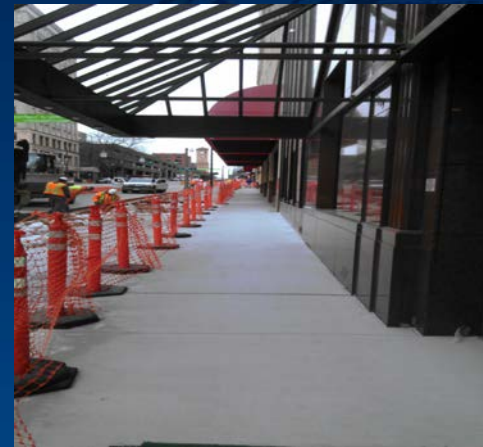
Pacific Avenue Streetscape
