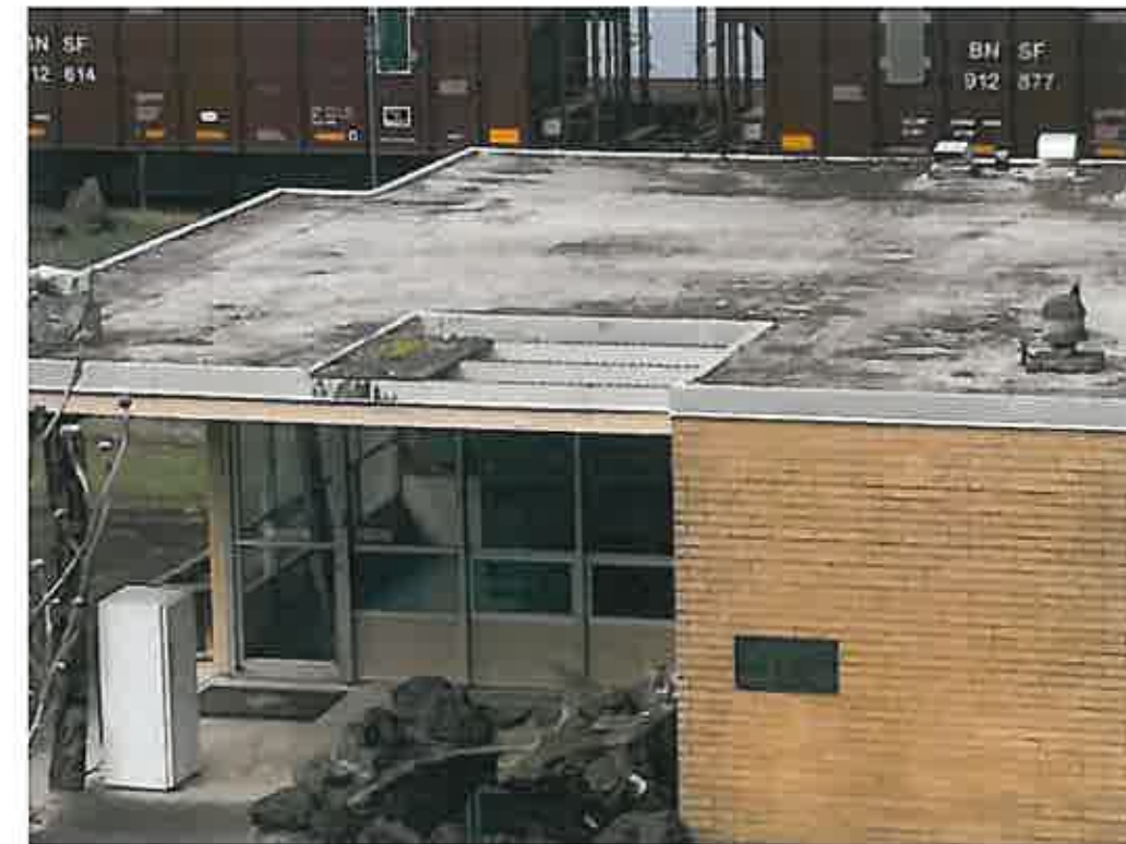
CITY OF TACOMA WESTERN SLOPES WASTEWATER TREATMENT PLANT: #2 OPERATIONS BUILDING ROOF REPLACEMENT ES14-0601S
