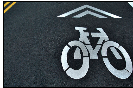
Shared Lane Marking
