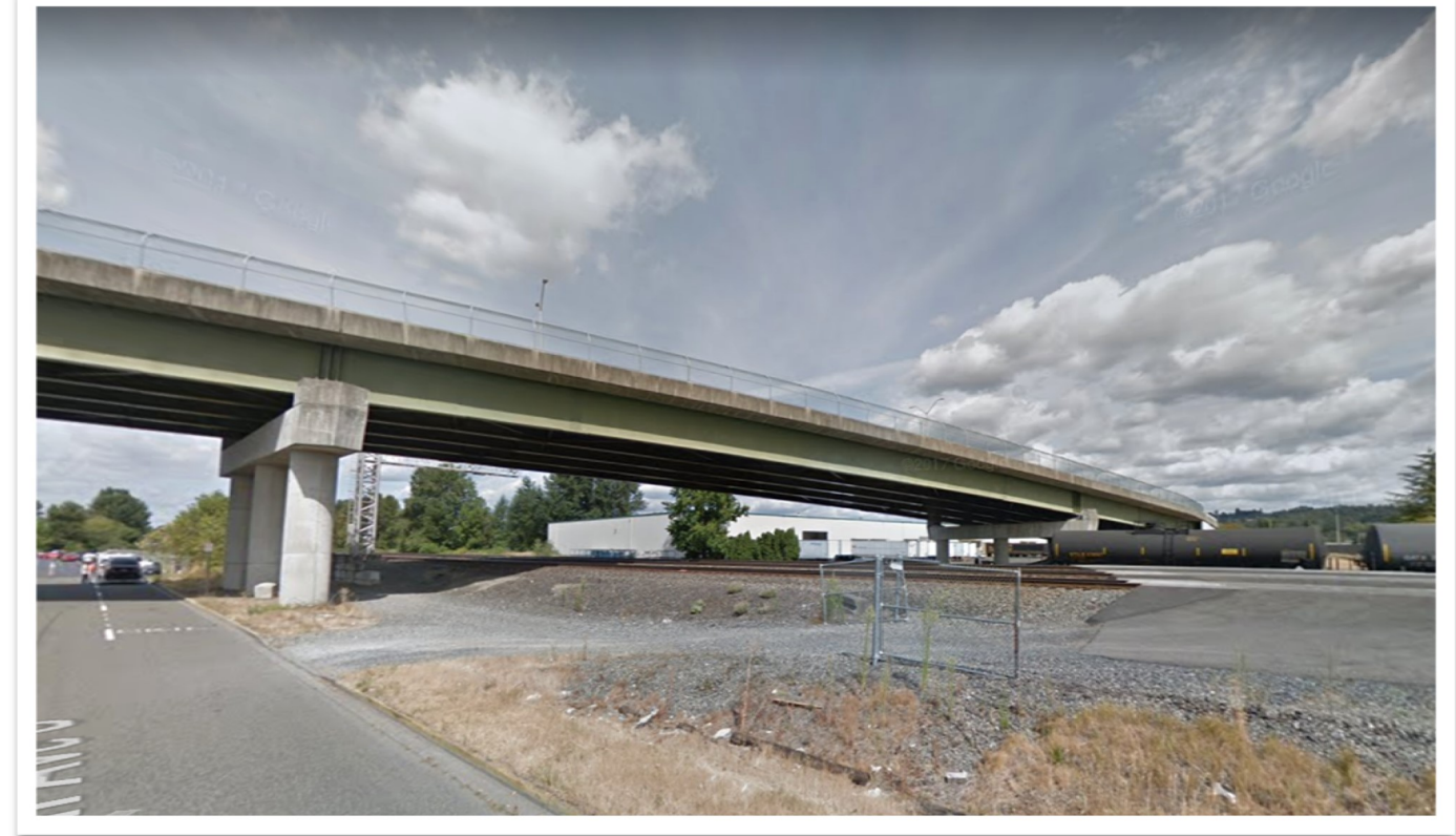
Example of a full grade separation.
