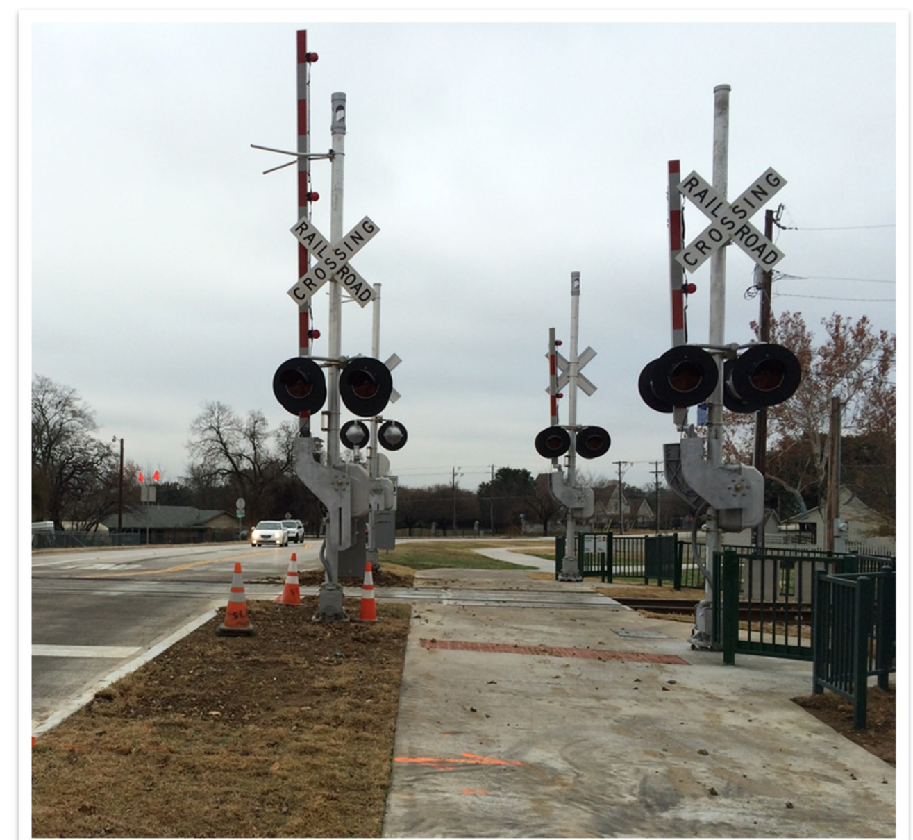
Example of vehicular and pedestrian gates.
