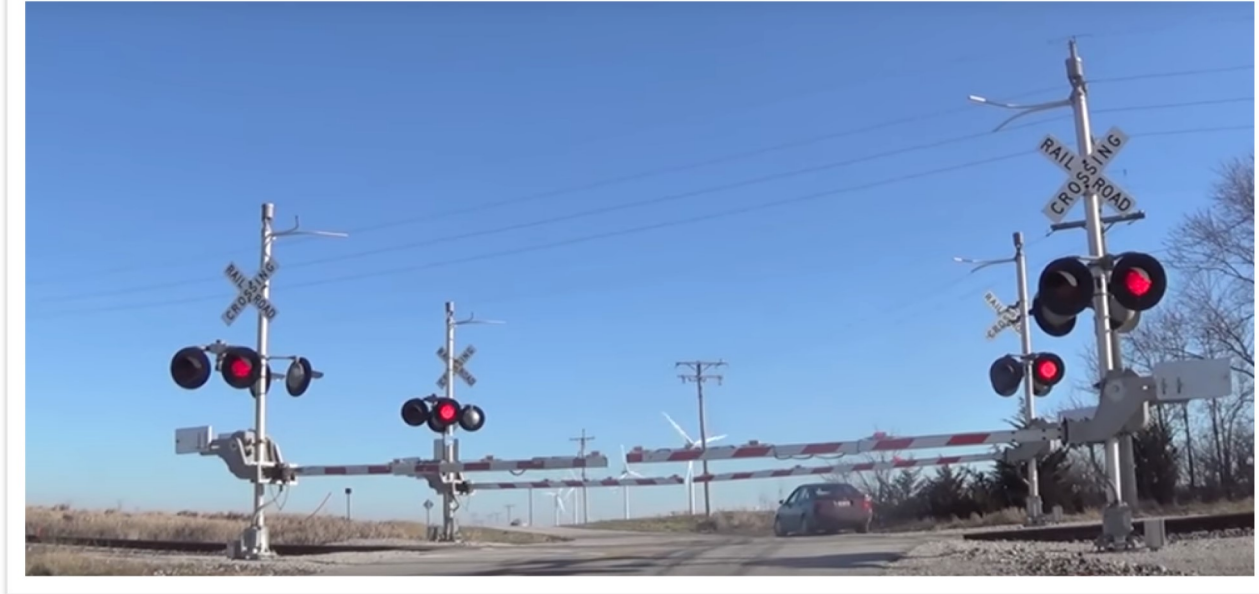
Example of 4 quadrant gates.
