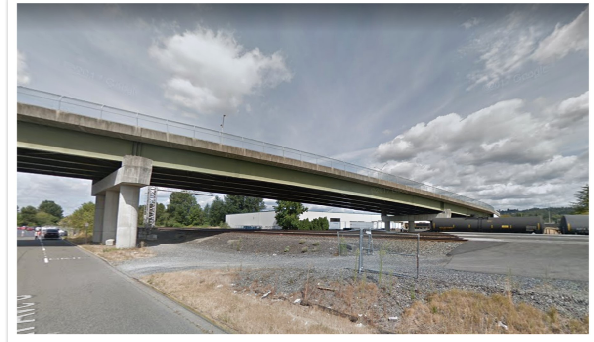
Example of a full grade separation.
