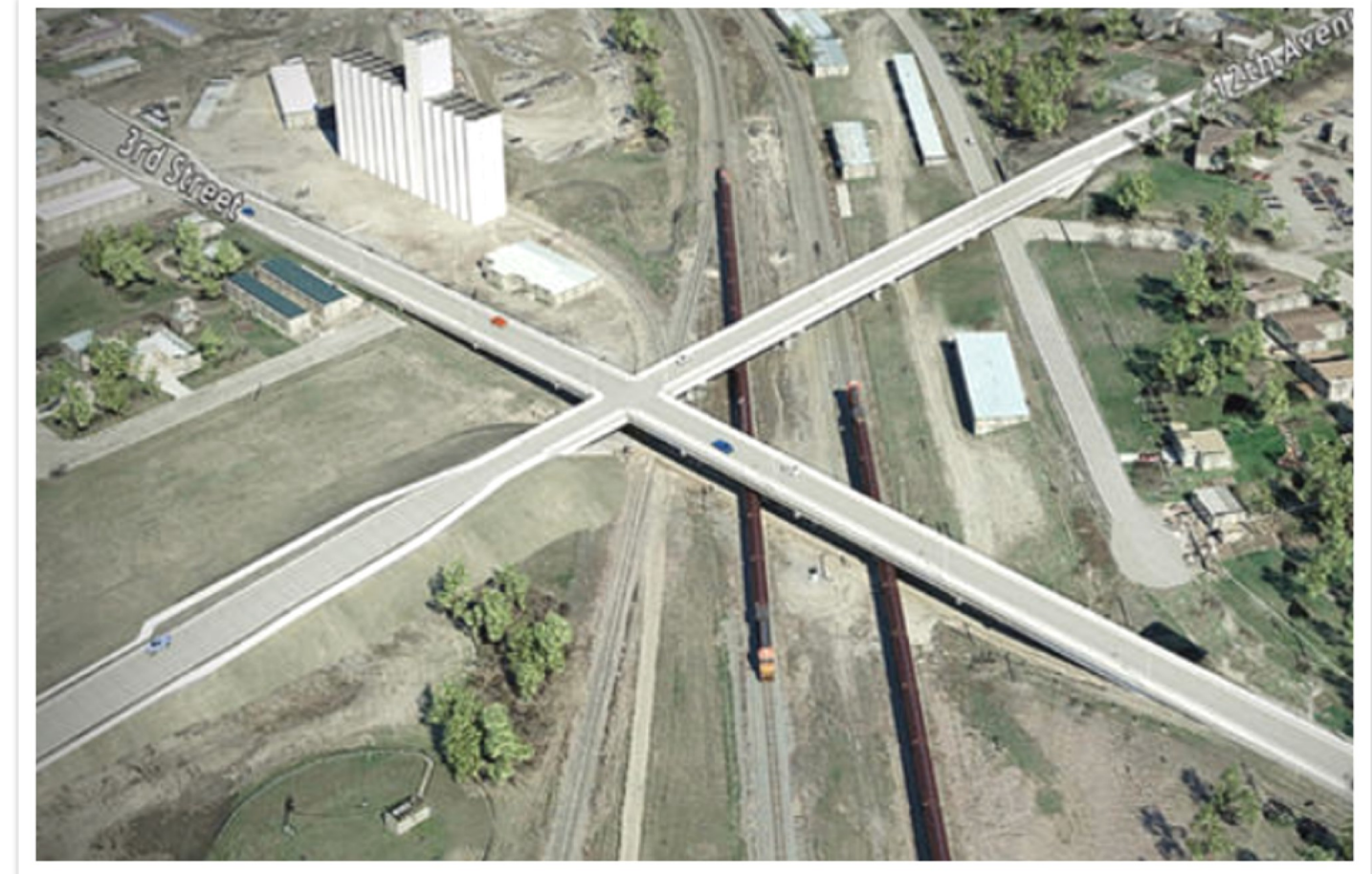
Example of a full grade separation.
