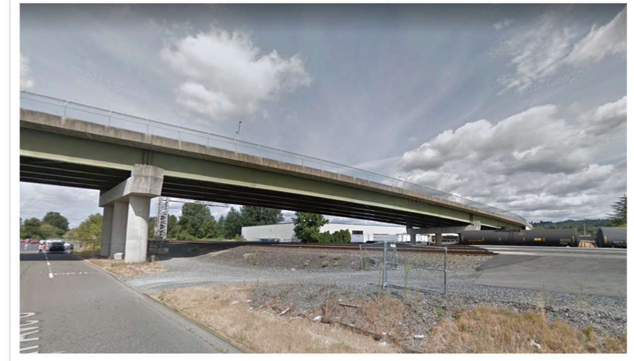
Example of a full grade separation.
