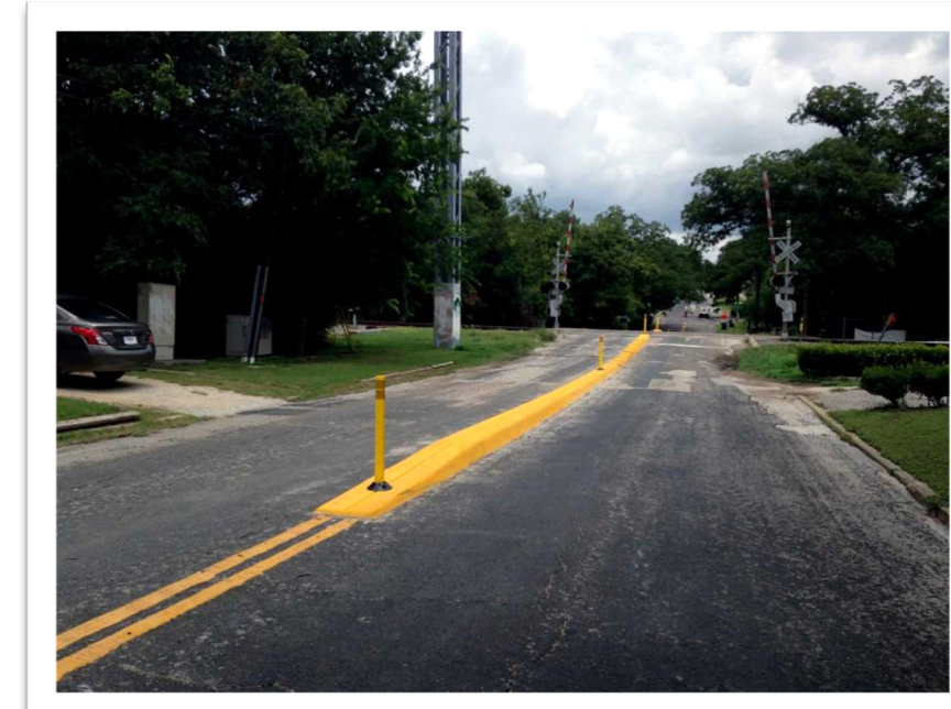
Example of a median in front of a railroad crossing.
