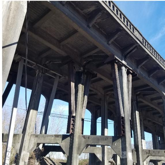
Spans supported by timber beams due to age
