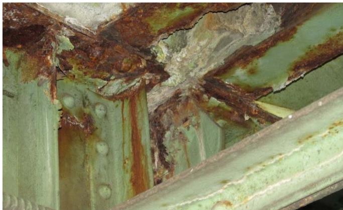
Localized heavy corrosion subject to repair
