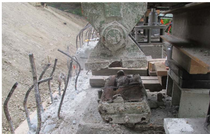
Replacement of frozen bearings at the settled south abutment
