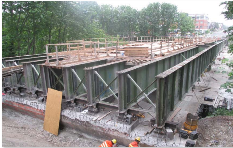
Bridge deck removed, south abutment wall removed, work deck can be seen under the girders
