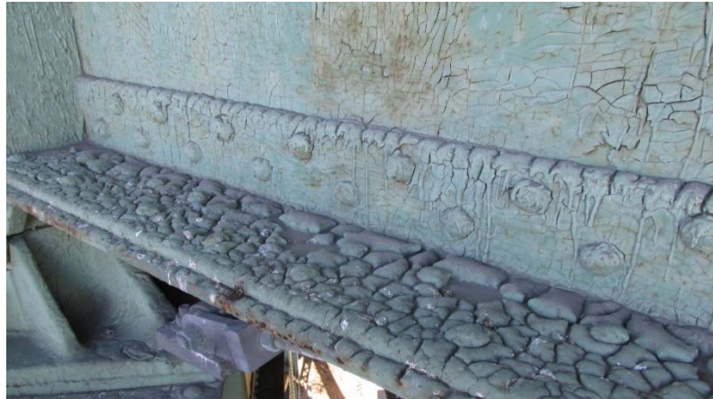
Carbonaceous fire-proof coating on steel girders
