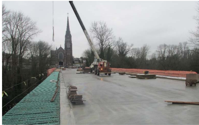
View of bridge deck constructed with light weight concrete looking south
