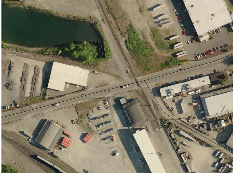
Figure 3 East Thea Foss Transportation Systems Conflict with Public Access Source: govME Map Tacoma
