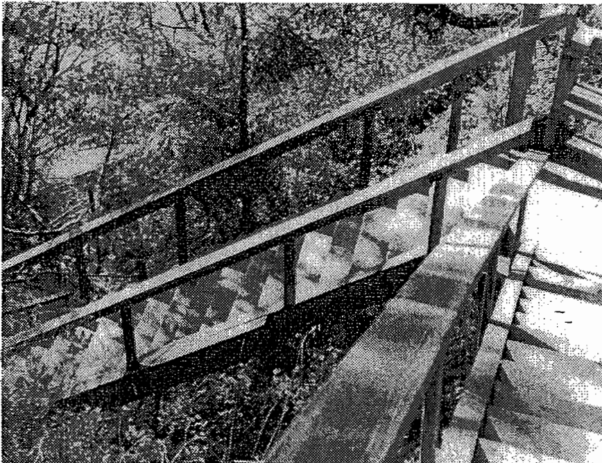
Stairs, such as these built on the slopes above Salmon Beach, can provide access down the steepest slopes without significant grading.
