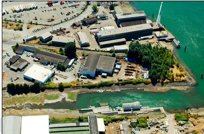
Figure 6 Under a plan accepted by the EPA, the Wheeler-Osgood and Thea Foss Waterways were cleaned. Approximately 425,000 cubic yards of contaminated sediments were dredged from the waterways and placed behind a containment berm in the nearby St. Paul Waterway. As part of the cleanup project, habitat restoration sites were constructed. In addition, wherever possible shorelines were enhanced to make them habitat friendly, including four areas along the Thea Foss Waterway. The Wheeler Osgood remains a potential site for further restoration. As shown in this image, native vegetation is lacking. Native plants along the shoreline would improve habitat functions.
