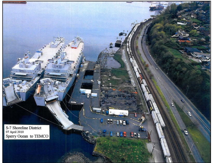
Figure 4 The image above shows a collection of creosote-treated pilings south of the Sperry Dock along Schuster Parkway. Removal of these pilings would improve water quality by removing a contaminant source. For decades marine piles were coated with creosote, a preservative that protected the wood from wood-boring organisms. Approximately 300 chemicals have been identified in coal-tar creosote, many of which have been found to be potentially toxic to fish, other marine organisms and humans.
