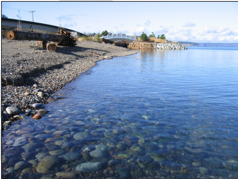
Figure 1 A beach restoration project was part of the development of Chinese Reconciliation Park along Ruston Way. The Project includes beach stabilization and restoration (addition of fish friendly substrate) as well as off shore restoration. The benefits include wave attenuation and reconnection of the shoreline and water, and enhanced nearshore marine habitat.
