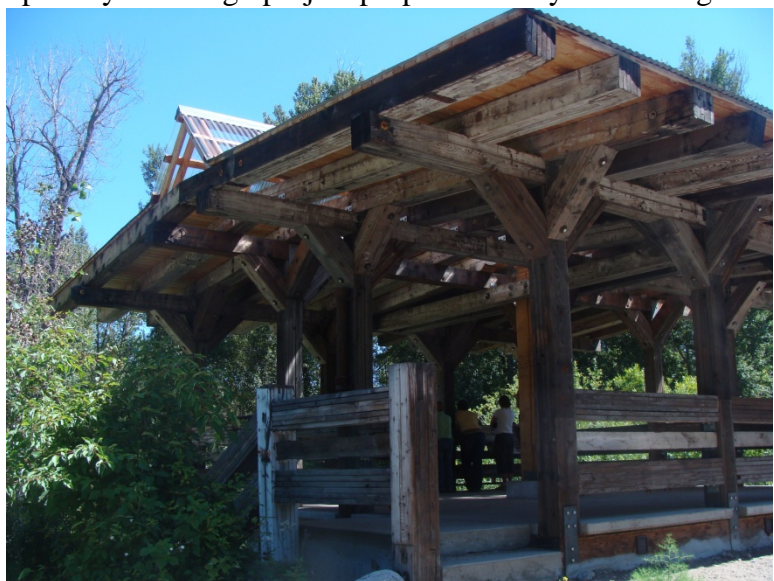
Figure 9-9: Viewing towers can provide visual public access at critical areas, industrial areas, and locations like this one on the Twisp River. Photo by Department of Ecology.
