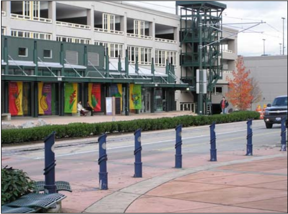
Photograph 1. Tacoma Dome Transit Station Source: Meadows Design Works
