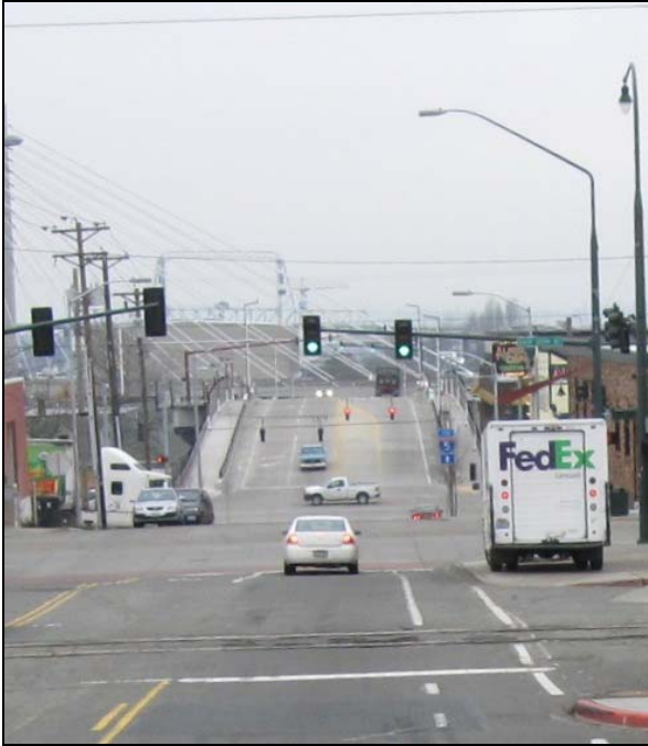
Photograph 3. East D Street Overpass (view north)
