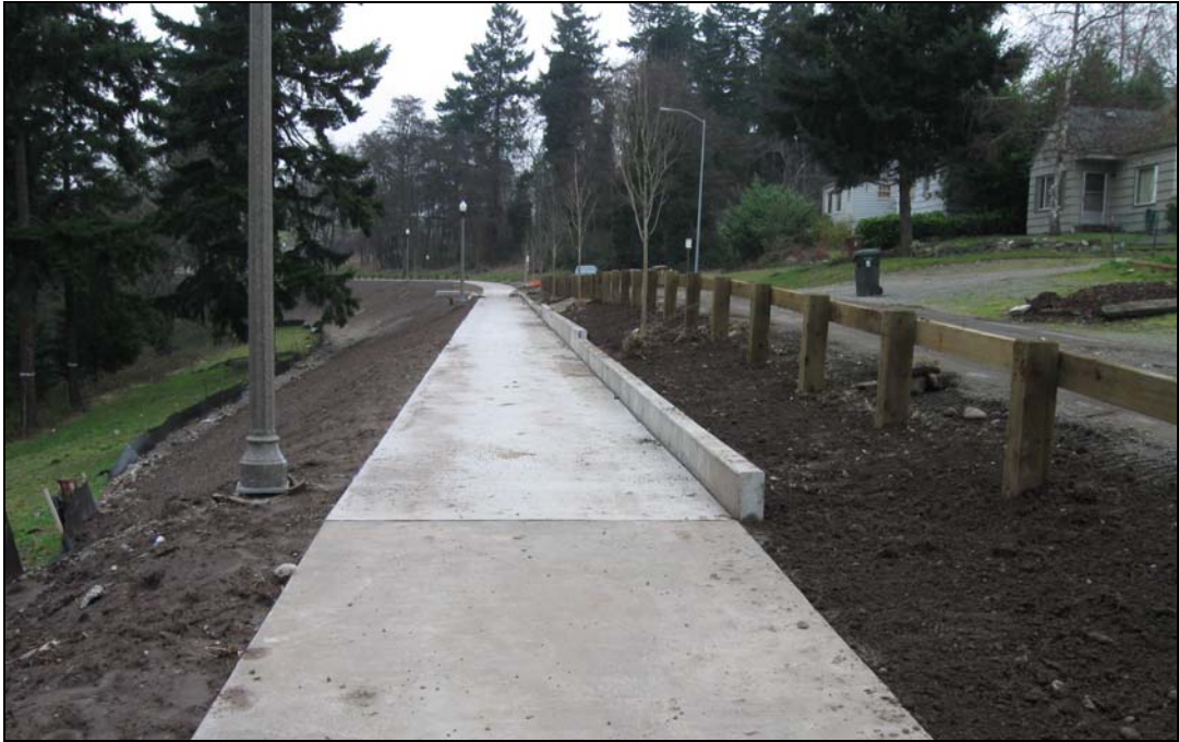
Photograph 8. McKinley Park – Path Currently Under Construction
