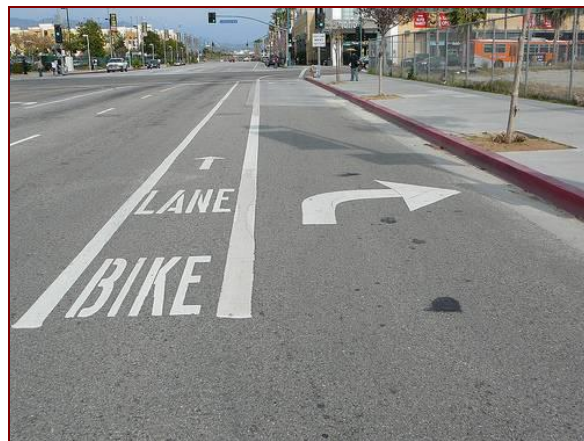
Continuing a bike lane straight while providing a right-turn pocket reduces bicycle/motor vehicle conflicts
