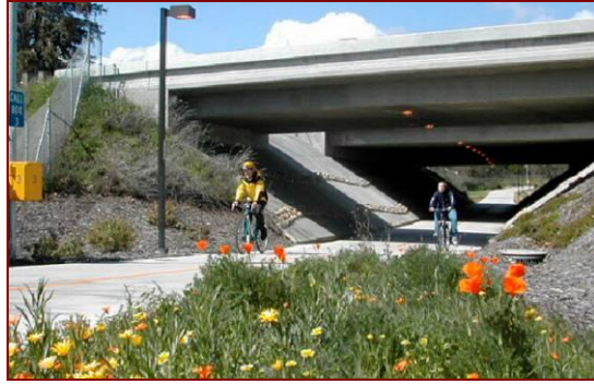
Type 4 Grade-Separated Undercrossing
