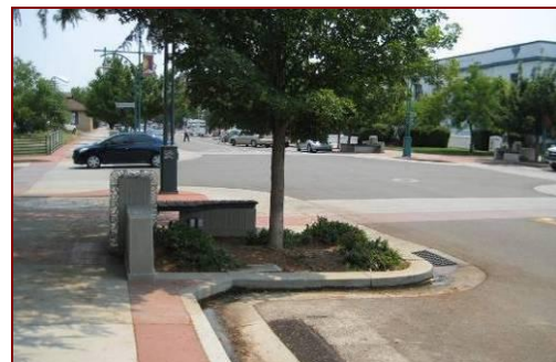
Curb bulb-outs can be a good location for pedestrian amenities, including street trees
