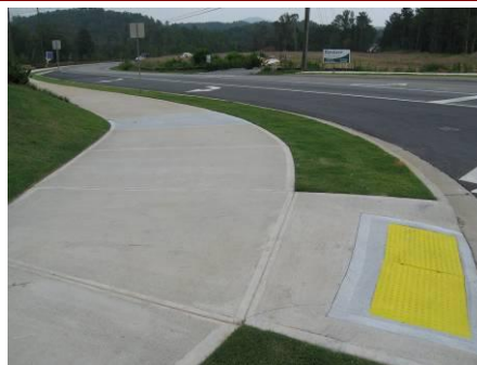
A diagonal ADA-compliant curb ramp
