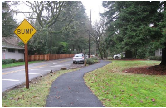
Asphalt is a common sidewalk surfacing material
