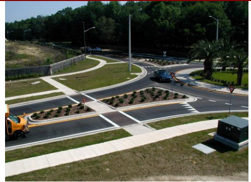
Modern roundabouts provide good pedestrian crossings in advance of the circle
