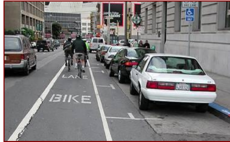
This bike lane provides parking “T’s” to minimize the danger of ‘dooring’
