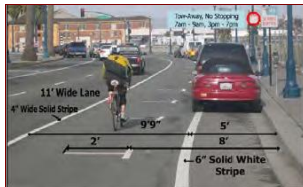
Floating Bike Lane when parking is allowed on The Embaradero, San Francisco
