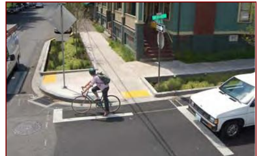
Bicycle forward stop bars encourage cyclists to wait to cross where they are visible to drivers
