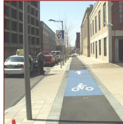
This cycle track in Cambridge, MA is separated from traffic by parking, light poles and grade
