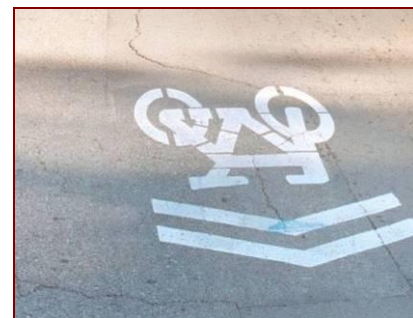
Shared lane marking
