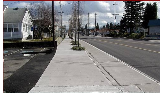
Concrete is often used as a shared-use path material, and also can be used for sidewalks
