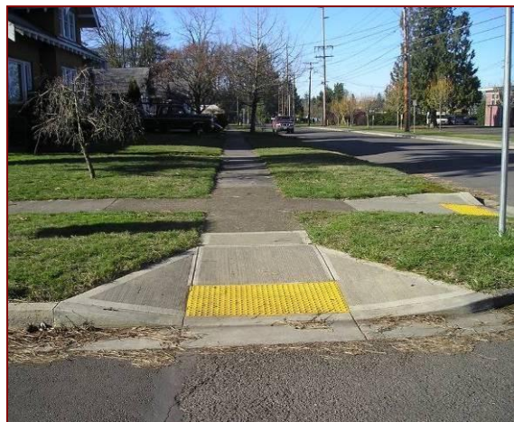
Example of an ADA-compliant perpendicular curb ramp
