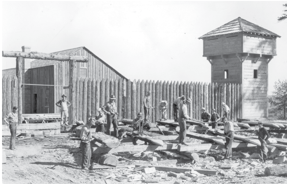
Fort Nisqually Restoration, Summer 1934 Fort Nisqually Collection
