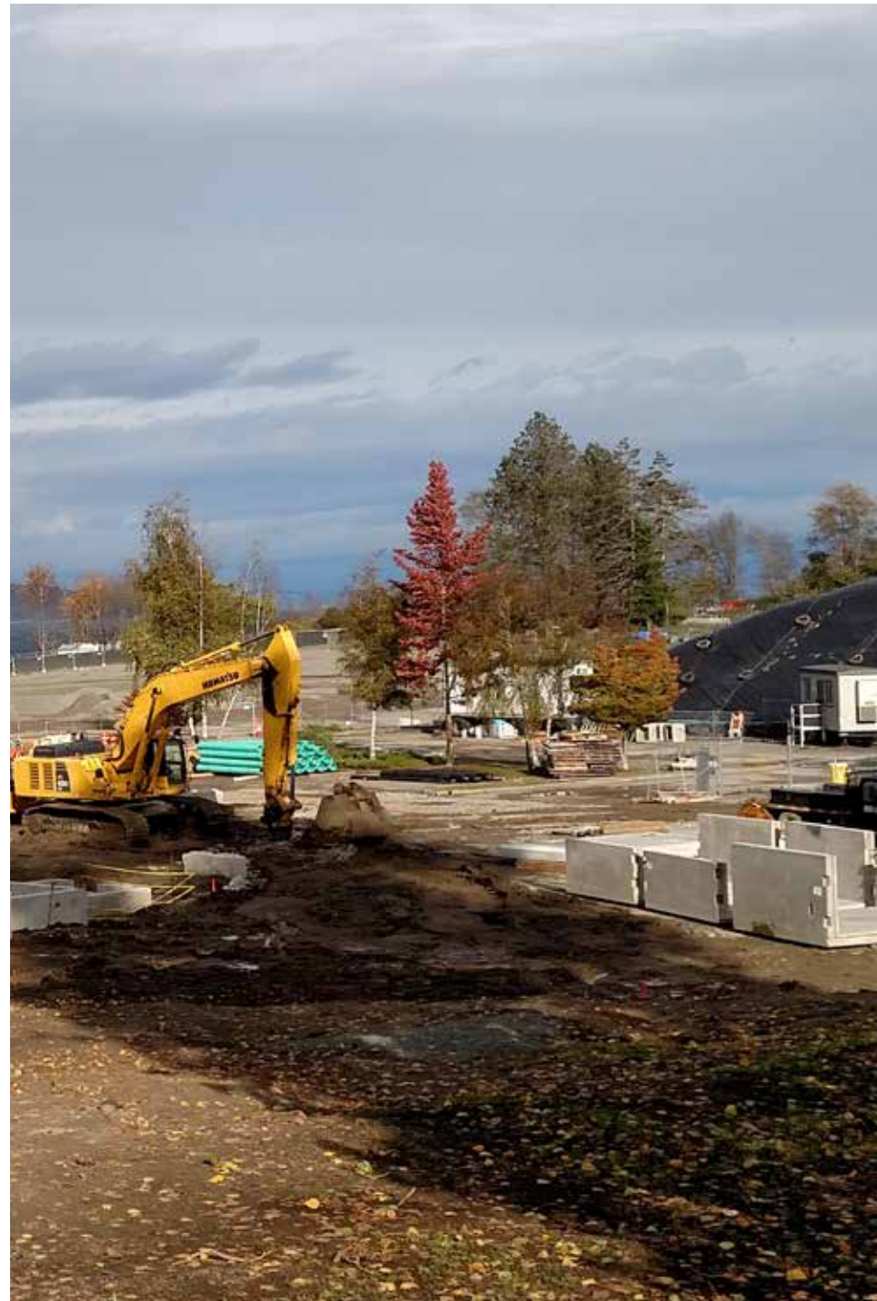
New Stormwater Facilities Being Installed at the Triangle
