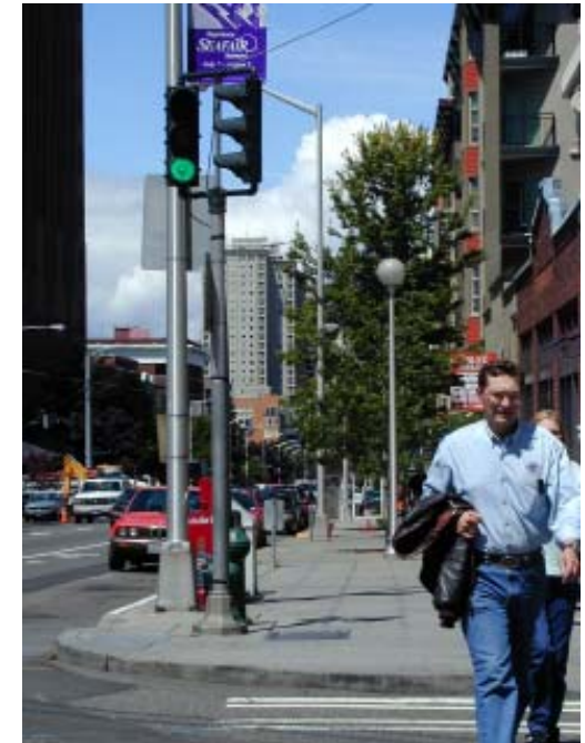
Post-top or side-mounted signals are more urban in character than large mast arms.
