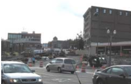
Convention Center site looking west from Pacific Ave.
