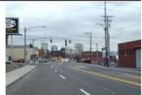
Jefferson St. between S. 21st and 23rd St. looking north.
