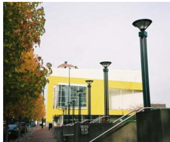
Contemporary pedestrian light used on Broadway Ave.
