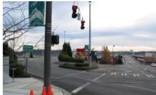
Existing gateway element at "A" St. intersection.
