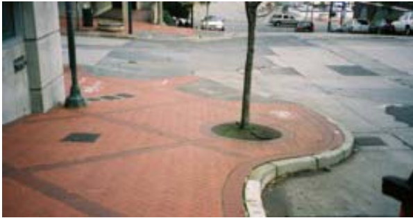
Brick paving is used as an accent on many downtown sidewalks and is appropriate where special paving is indicated.
