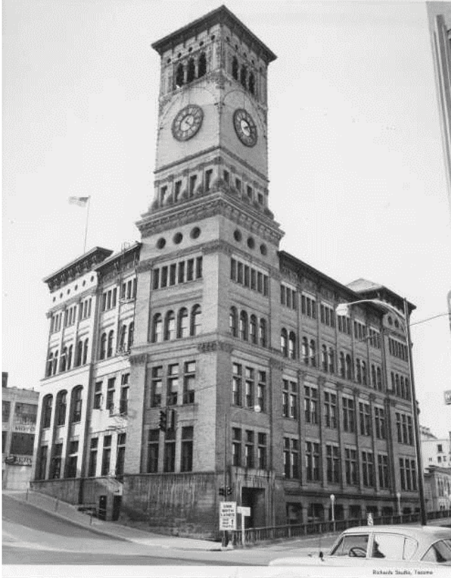
FIG. 5-26 Built in 1892, Old City Hall served as the seat of Tacoma’s government for 70 years. Periods of subsequent abandonment earned it a place on the WA Trust for Historic Preservations’s Most Endangered Properties List in 2011.
