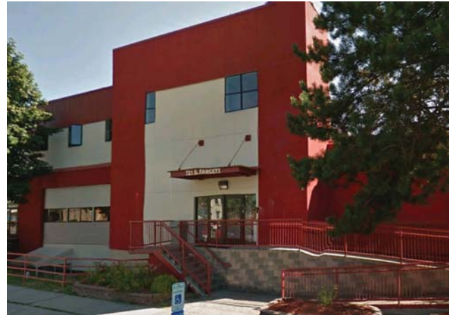
FIG. 6-7 Metropolitan Development Council housing at 721 South Fawcett Street.
