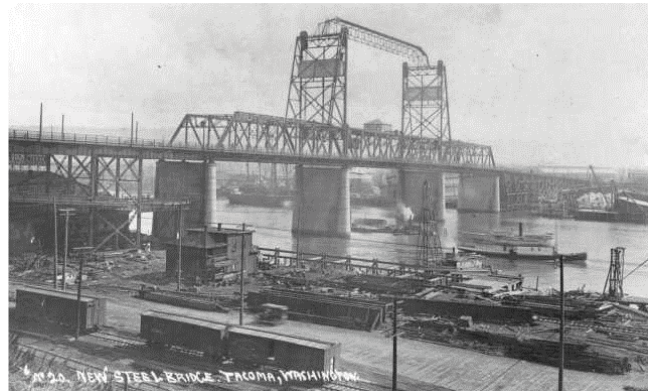
FIG. 5-24 The 11th Street Bridge (later named the Murray Morgan Bridge to honor the local historian) opened on February 15, 1913. The 2,100 foot steel bridge connected the Tideflats to the downtown business district and allowed larger ships to traverse the City waterway.
