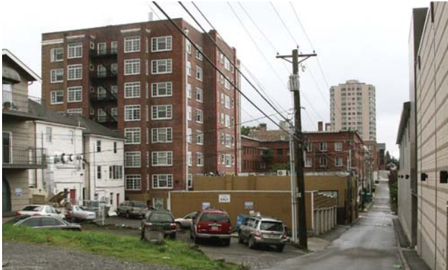
FIG. 2-6 The Stadium district is home to a variety of multifamily housing options, including condos as well as rental units.
