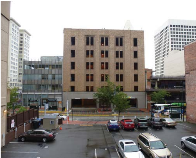
FIG. 2-17 A view from Broadway east toward structured and surface parking flanking Commerce Street.
