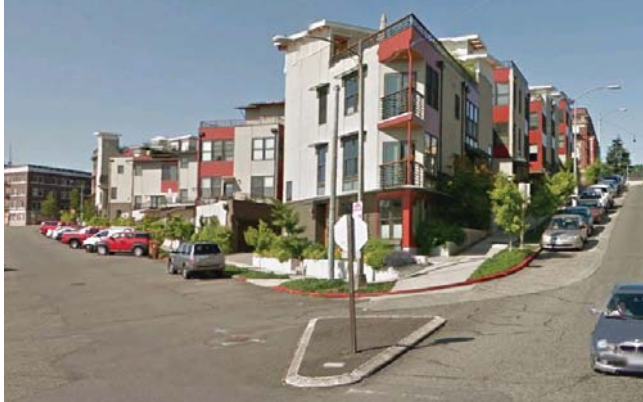
FIG. 2-8 The Triangle Townhomes, a 27-unit condo development in the St. Helens district, is one of the first Built Green projects in downtown Tacoma.
