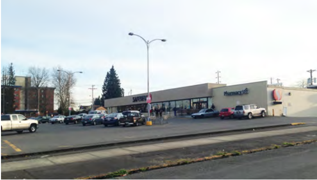
FIG. 7-20 The surface parking lots surrounding the Hilltop Safeway, a key community asset, have the potential to be developed with infill projects that could provide additional housing and commercial activity.
