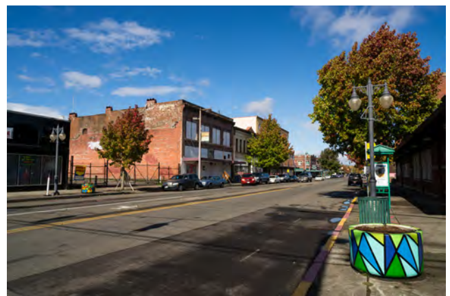
FIG. 5-4 Pedestrian infrastructure along Martin Luther King, Jr. Way: painted planters, information kiosks, and pedestrian-scaled street lights.
