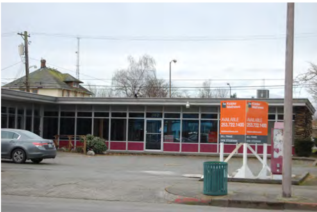
FIG. 3-4 Although Hilltop's business district has experienced an economic resurgence in recent years, many vacant storefronts remain.
