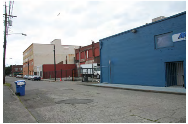
FIG. 5-2 The neighborhood's streets are in various states of repair.
