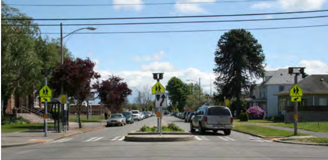
FIG. 2-18 Crosswalk improvements near McCarver Elementary School.
