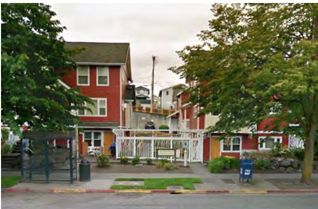
FIG. 3-12 The Matsusaka Townhomes, a subsidized family housing development on South Yakima Avenue.
