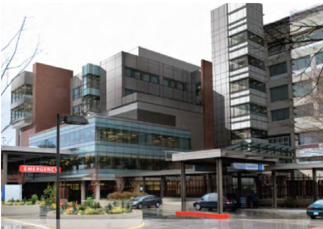
FIG. 7-4 Two new floors were added to the Milgard Pavilion on the MultiCare healthcare campus as part of a multi-phase strategy for expanding women and children's services.
