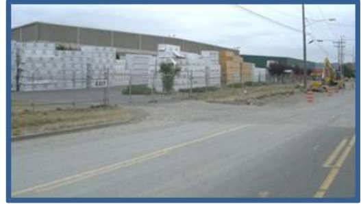
Roadway under construction
