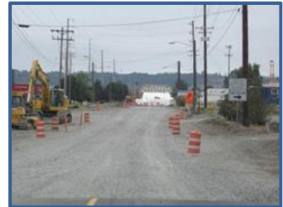
Roadway construction in the port area
