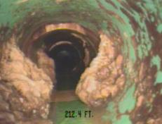
Moderate debris/grease described as reducing the pipes capacity by 25 to 50 percent.
