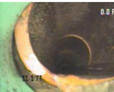
Moderate offset joint May cause some buildup of debris but Has a more likely chance for causing a typically would not cause a backup and backup over time and exposes the soil the joint.
