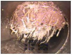
Severe root intrusion Severe root intrusion, obstructing 50 percent or more of the pipe, is either already having an impact on the working function of the side sewer or soon will be.
