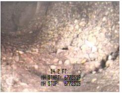
Severe exposed aggregate with holes Pipes that have severe exposed aggregate resulting in holes and missing walls of the pipe are considered to have reached full structural failure even though flows may still be able to travel through or seep out of the pipe. Pipes of this severity will eventually fully collapse which may cause severe debris to settle in, sewer backups and possibly sinkholes.
