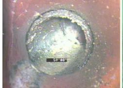
Minor offset joint Unlikely to cause a buildup of debris and typically doesn't cause any negative effect on the sewer.
