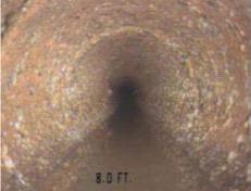
Moderate exposed aggregate Moderate exposed aggregate that covers the full circumference of the pipe likely is not affecting the working condition of the side sewer but the structural stability of the pipe is decreasing. Once full aggregate is showing, it is very difficult to tell how much pipe wall thickness remains. Pipes in this category may be good candidates for rehabilitation prior to them reaching full structural failure.
