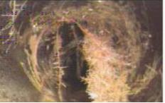
Moderate root intrusion Moderate root intrusion may or may not affect the working condition of the side sewer and will likely increase in severity over time. Roots that are blocking 25 to 50 percent of the pipe
