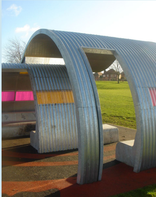
Coleshill Shelter completed
